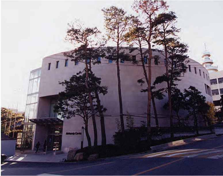
Artsonje Centre, Seoul, 2004 Architect: Jong-Sung Kim Photograph: Artsonje Centre
