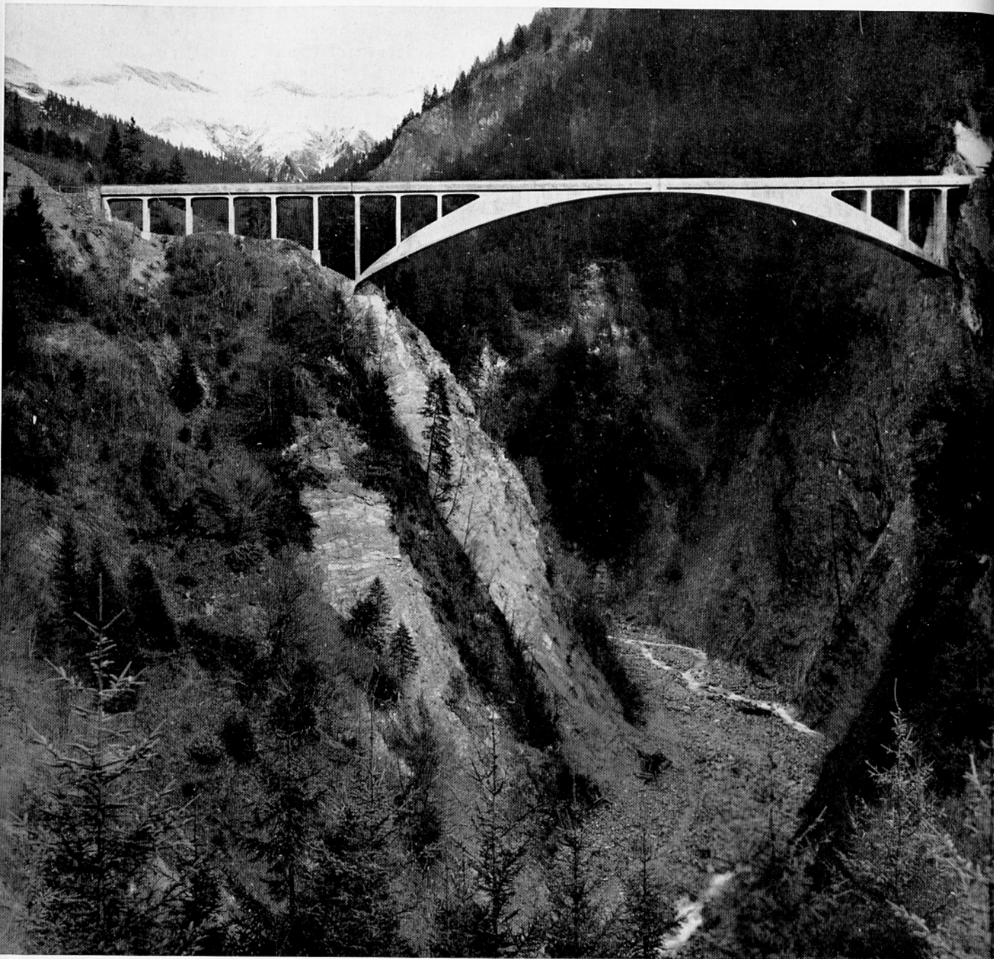
The Salginatobel Bridge in the Engadine, constructed 1929-30 (span: 90 metres). Robert Maillart, engineer. Photo: P. Morton Shand.
