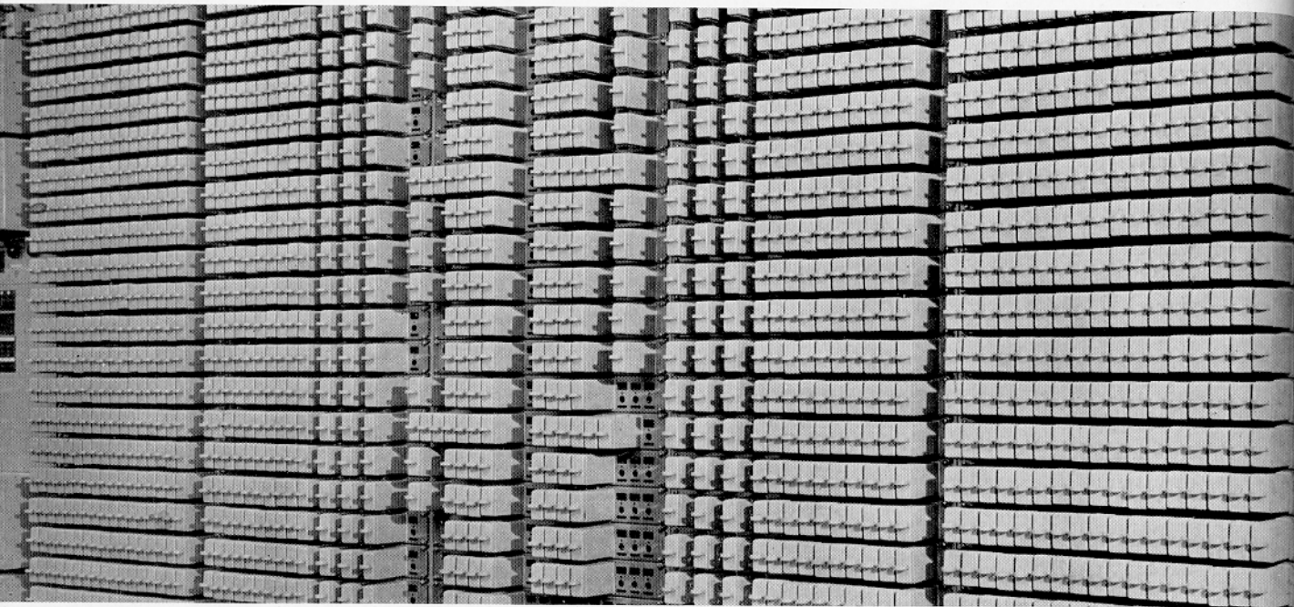
An architectural sense of design exemplified in an assembly of engineering units. The "B" Amplifier Output Switching Relays at Broadcasting House, London. Photo: B.B.C. copyright.
