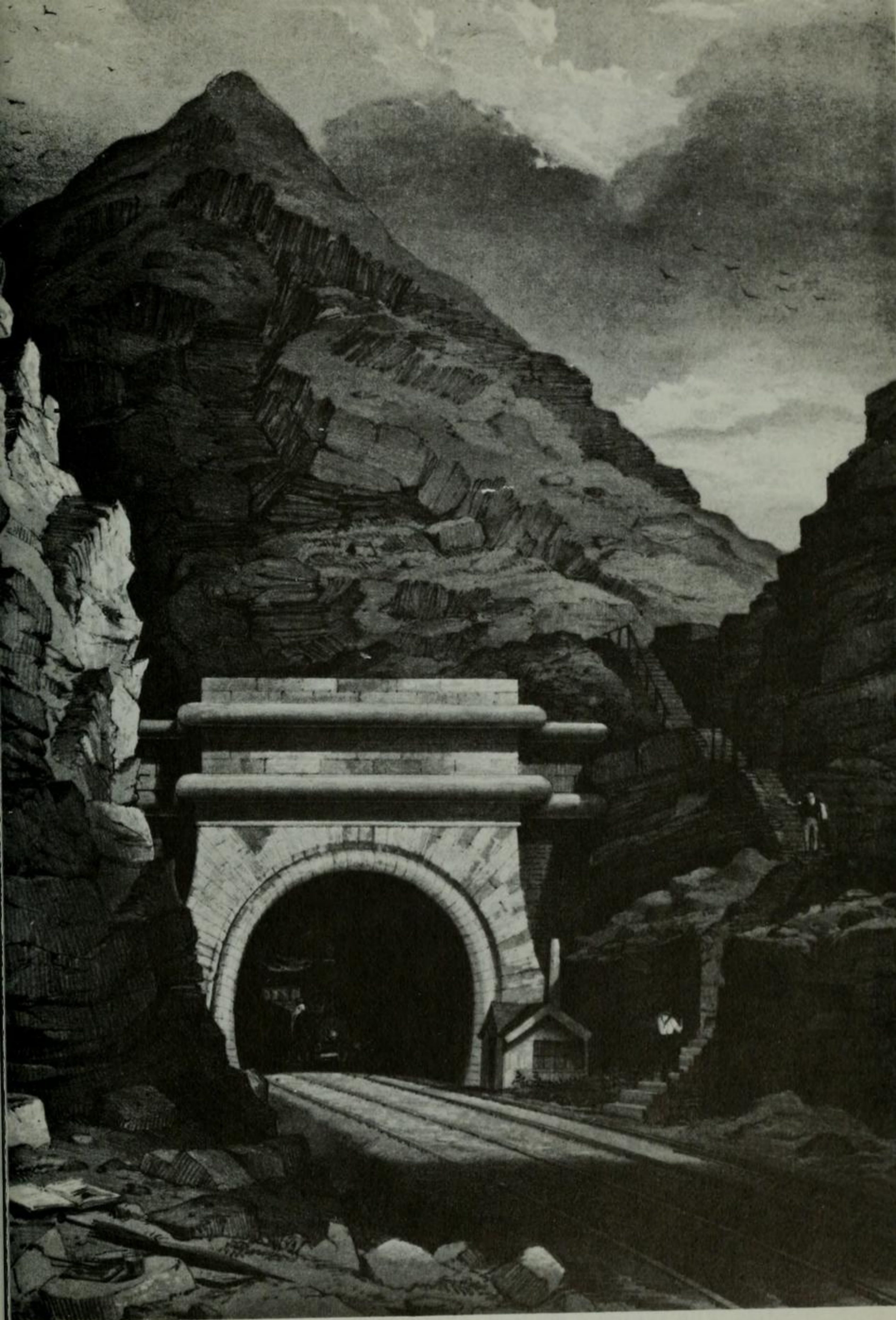
90. Summit tunnel, Manchester and Leeds railway, A. W. Tait.
