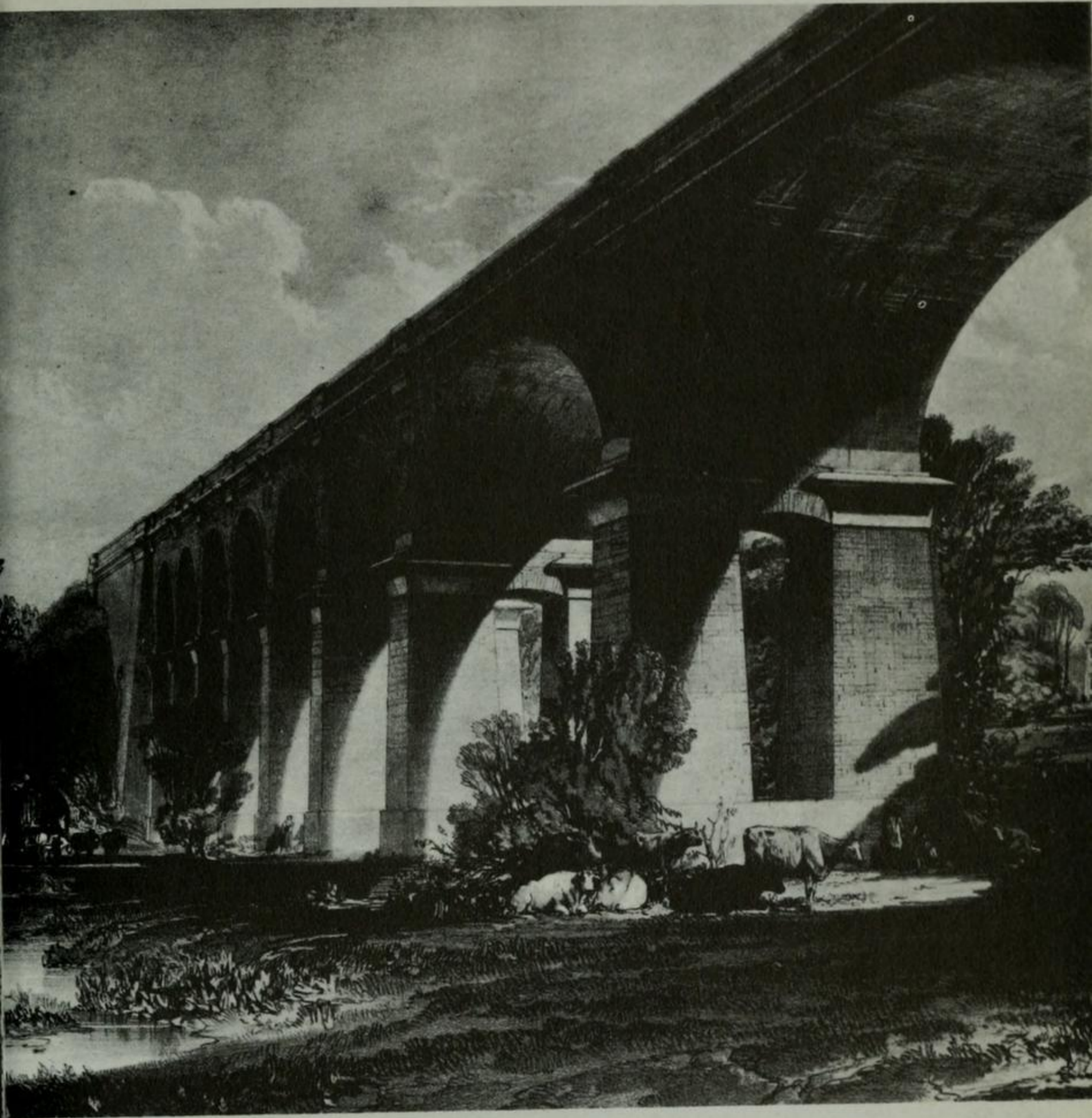
92. The Wharncliffe viaduct, Great Western Railway, J. C. Bourne.
