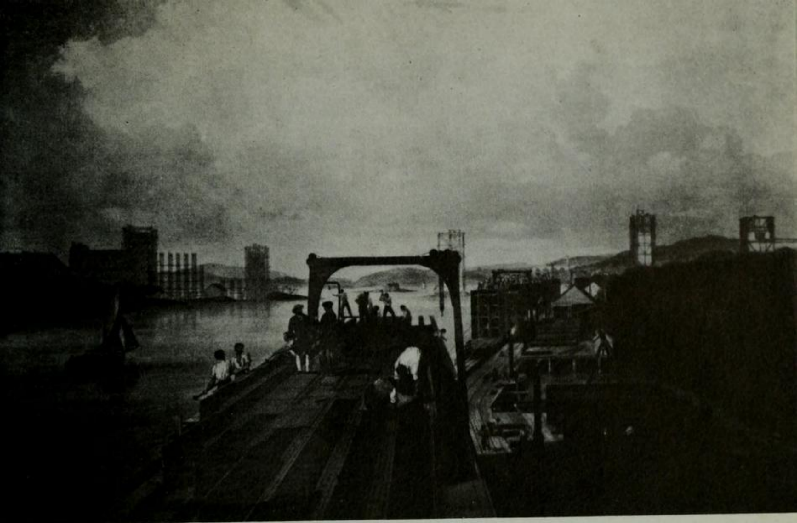
95. Britannia tubular bridge over the Menai Straits, 1849.
