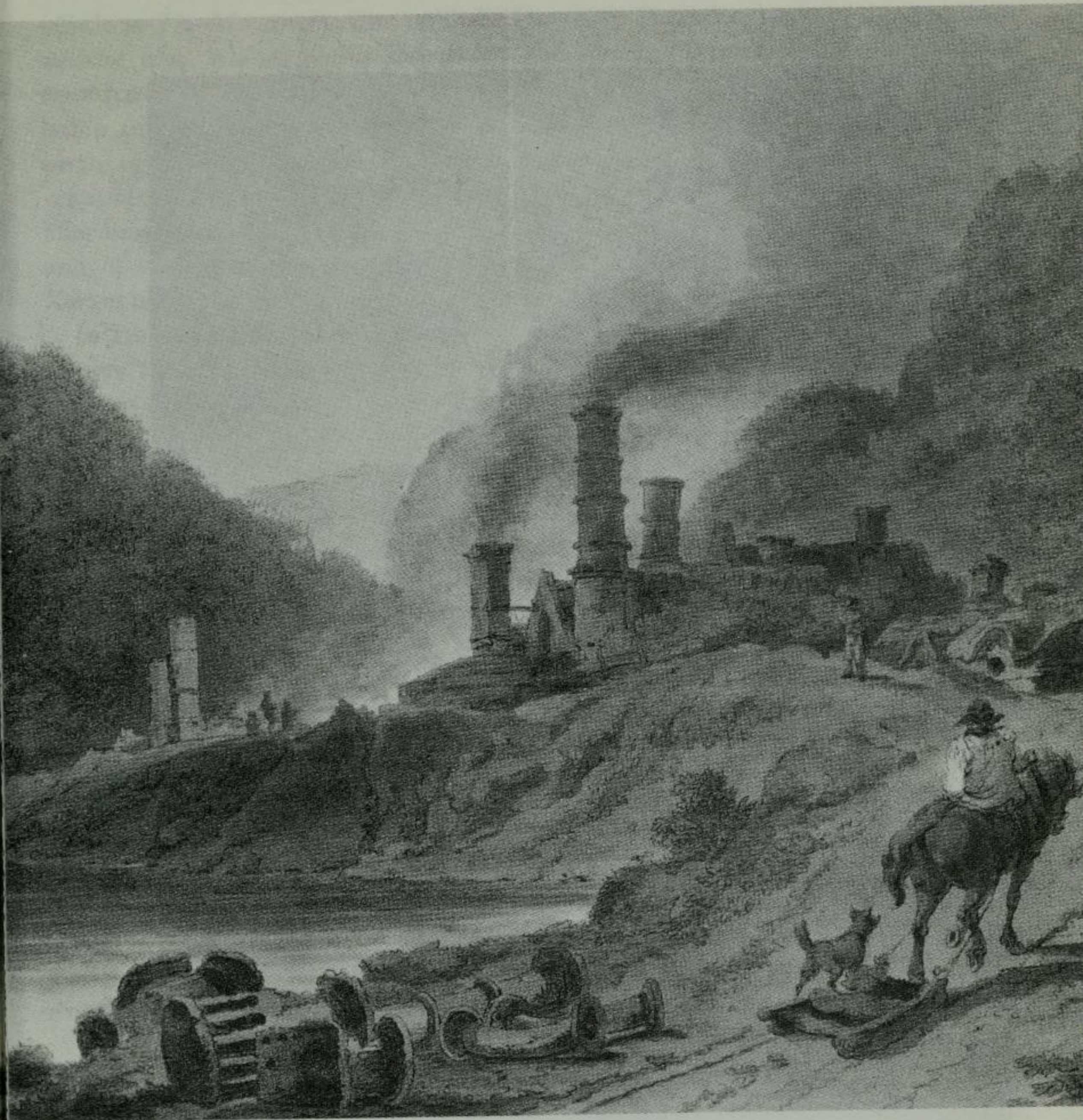
V IRON WORKS, COLEBROOK DALE (1805) after de Louthembourg
