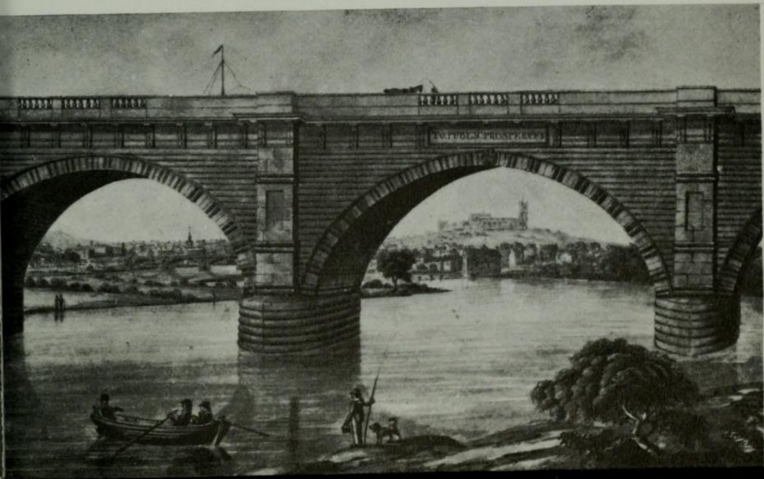
37. The Lune Aqueduct, c. 1798.
