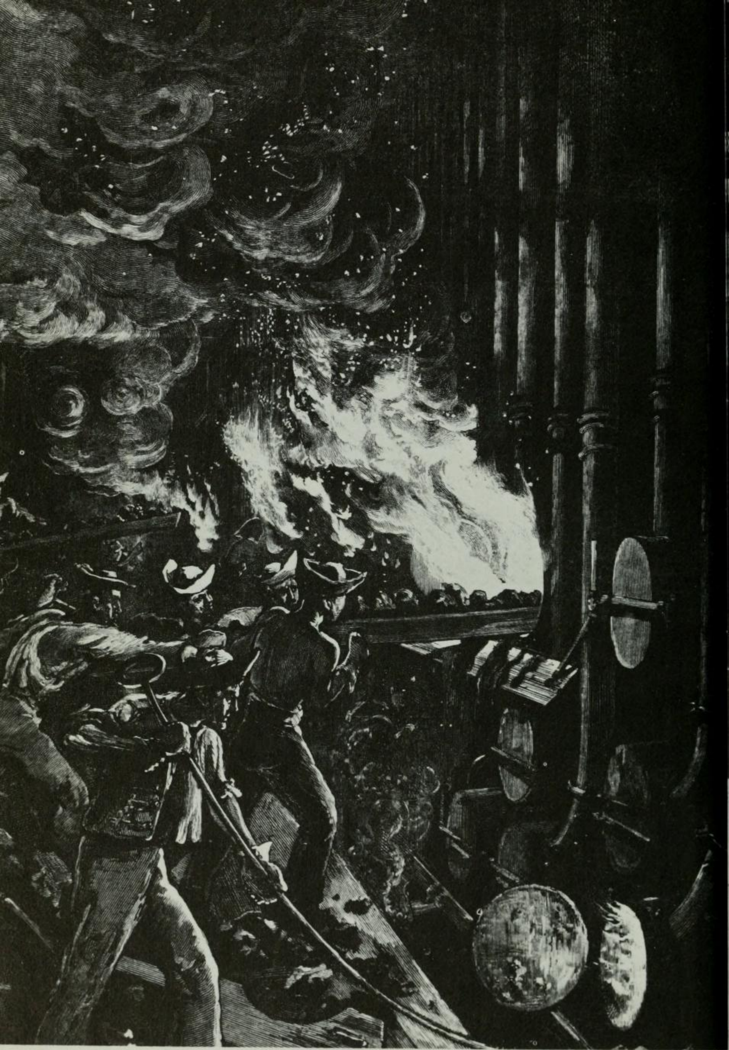
111. Charging retorts at the Beckton gasworks, 1878.
