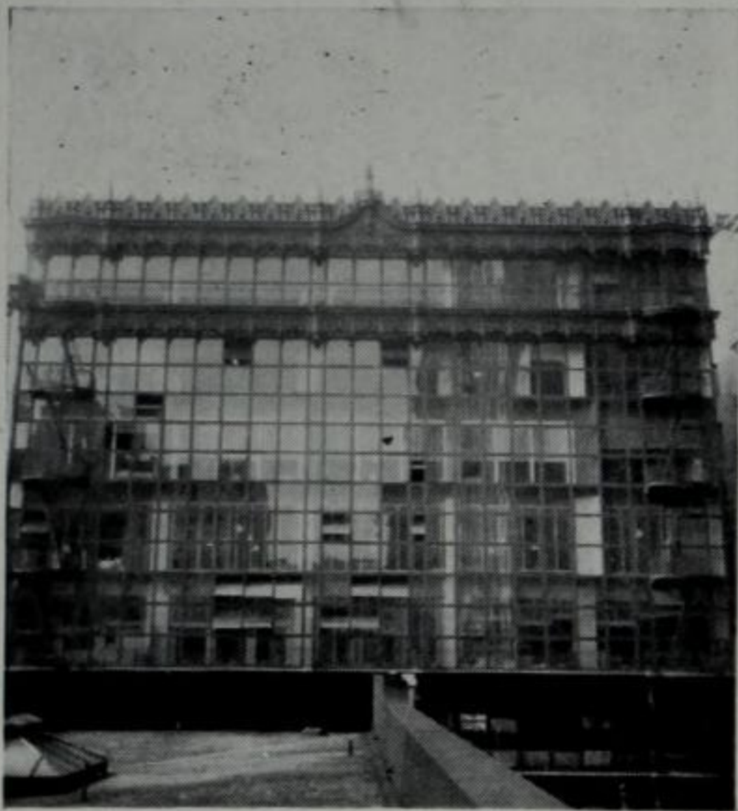
Fig. 131. W. Polk, 1916 This building in San Francisco shows a complete glass facade. Except for "gingerbread" on the top, it could be the pride of any contemporary architect
