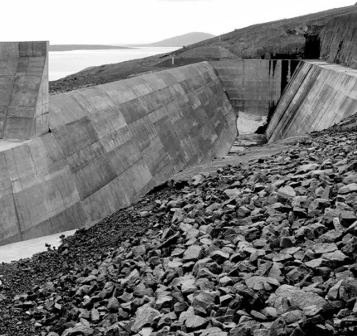
Kárahnjúkar hydroelectric dam in the eastern highlands of Iceland. Photo: Pavel Mirkus
