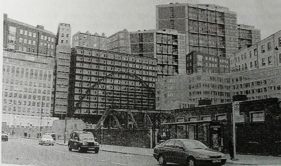
fig.7 A Variety of Housing Introduced to Liverpool Street
