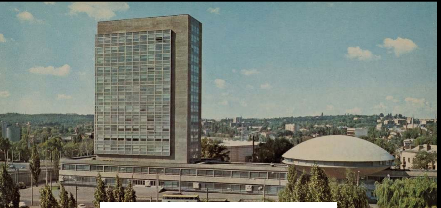
THE UKRSSR INSTITUTE FOR SCIENTIFIC AND TECHNICAL INFORMATION AND TECHNICAL-ECONOMIC RESEARCH FOR THE STATE PLANNING COMMISSION. ARCHITECTS: LEV NOVYKOV AND FLORIAN YURIEV. 1971. POSTCARD. PHOTO: I. KROPYVNYTSKY.
