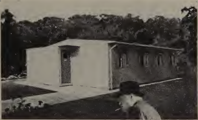
20. "Churchill House." Model of an English steel constructed dwelling to be manufactured after the war in numbers of 300,000. Such a procedure in prefabrication, repeating in great numbers the same type of house, is too rigid and too dull.
