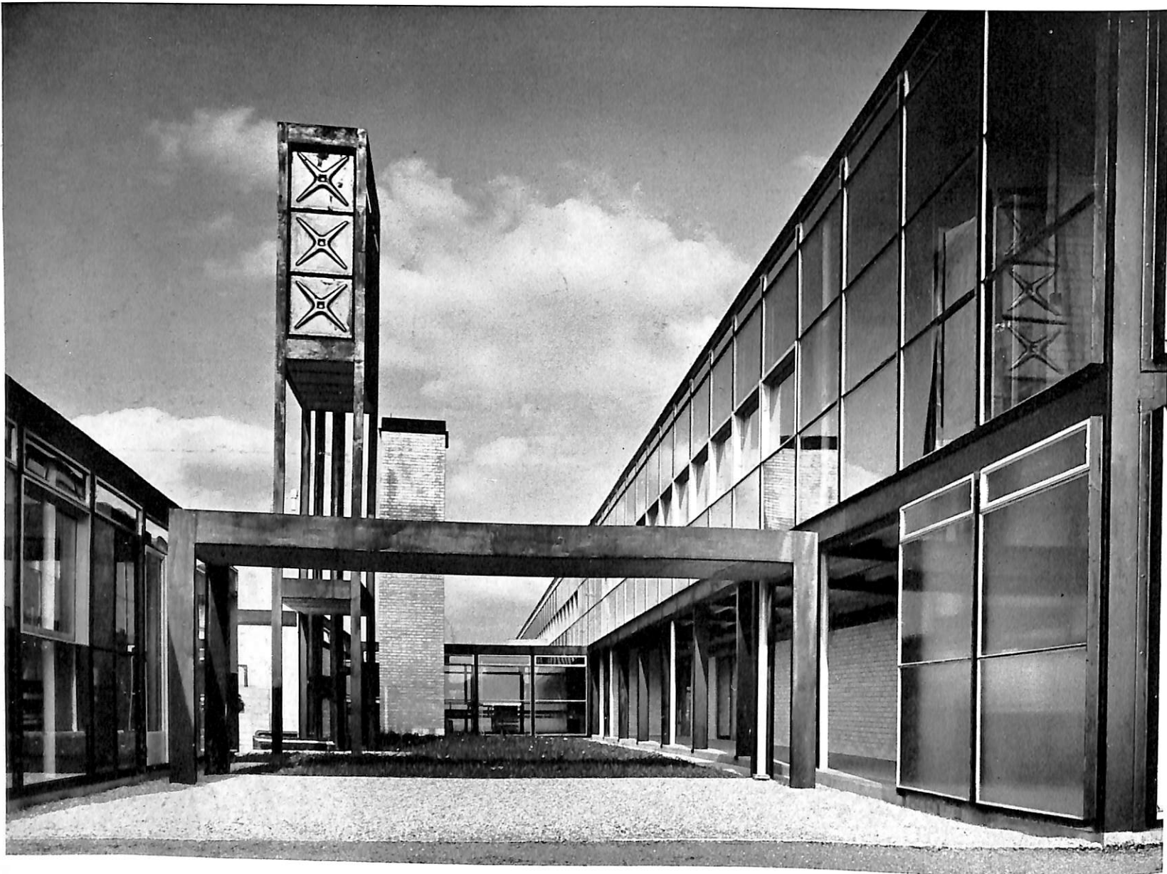
31 Water-tower and service rooms
