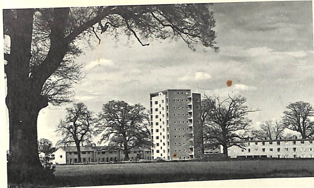
4 Frederick Gibberd; Harlow New Town (England), Housing at The Lawn, 1952
