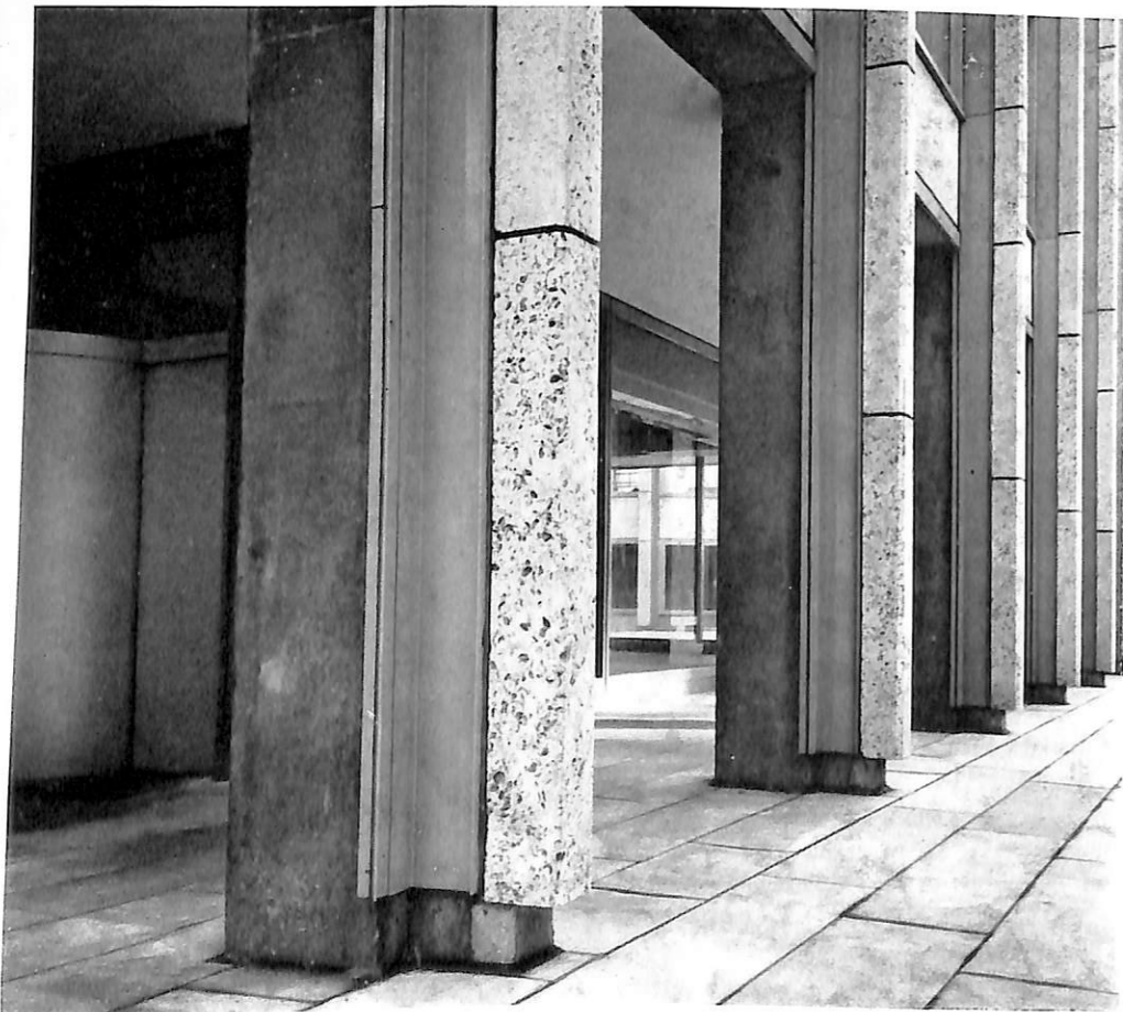
300 Detail of columns in piazza
