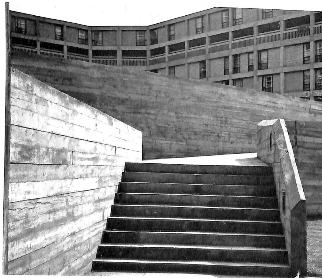
294 Steps and retaining walls in upper courtyard
