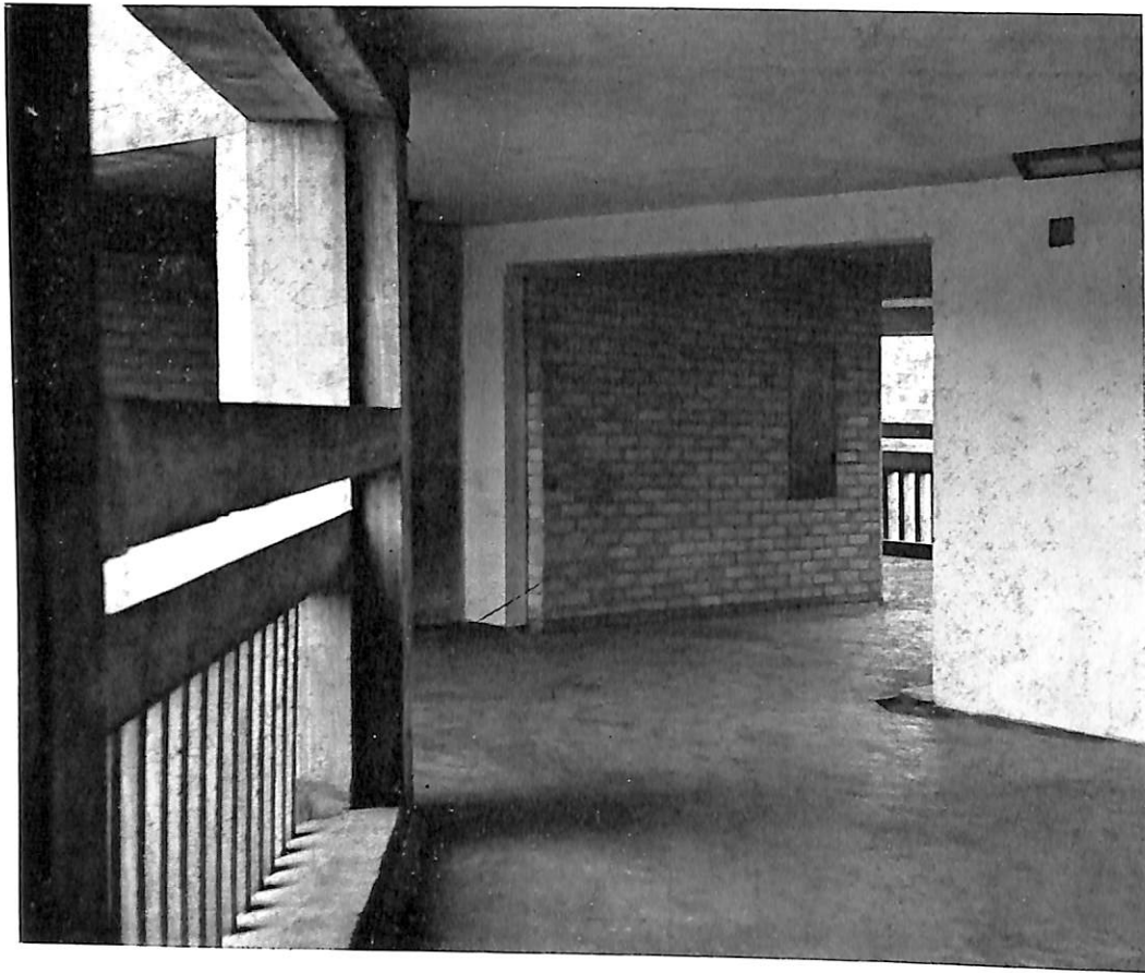
293 Street-deck passing through block
