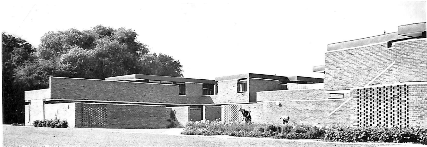
221 - 224 Sheppard, Robson and Partners; Cambridge (England), Churchill College, Fellows' Flats, 1960 221 Exterior
