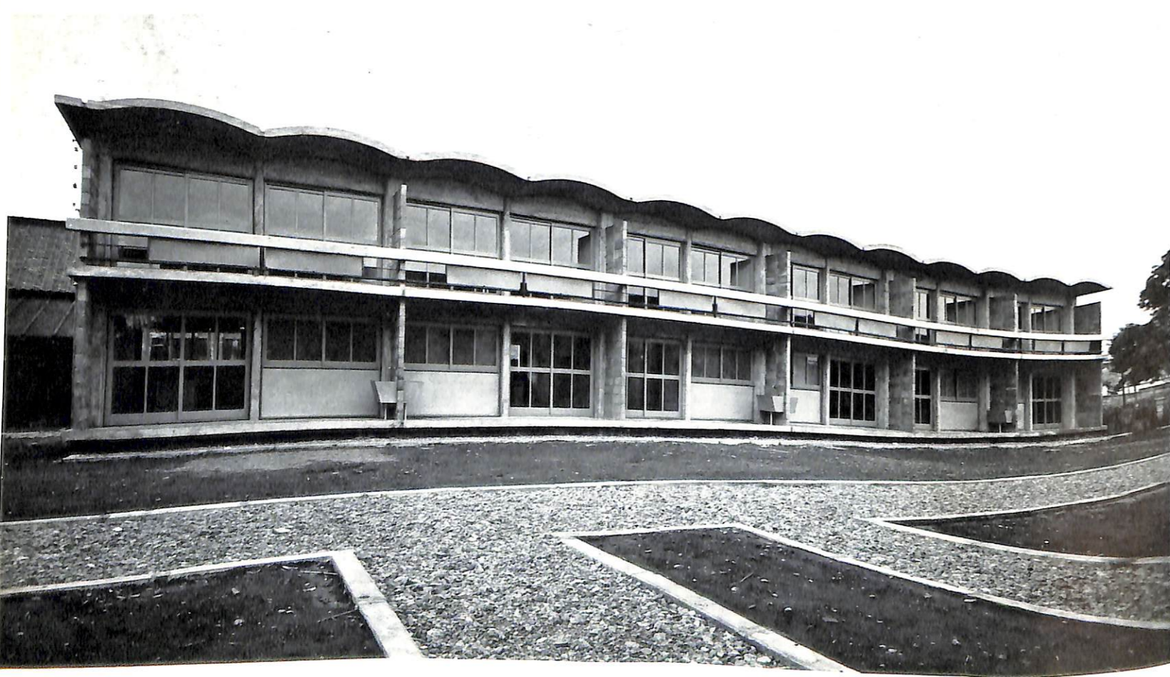
275 Courtyard elevation of main block
