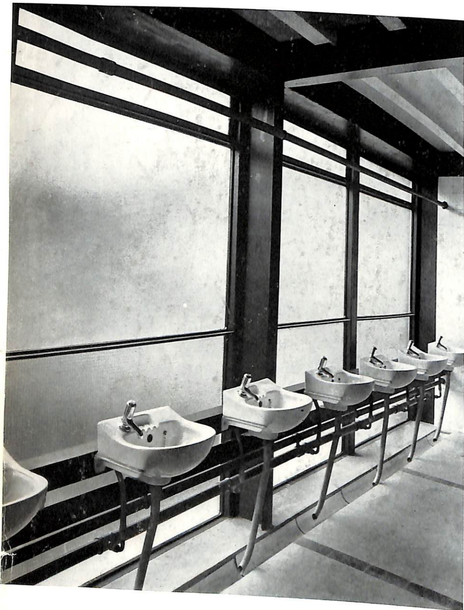
41 Washbasins in cloakroom
