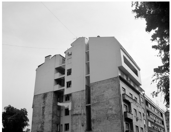
Roof extension in Belgrade photo by Sanja Stojanović, 2007
