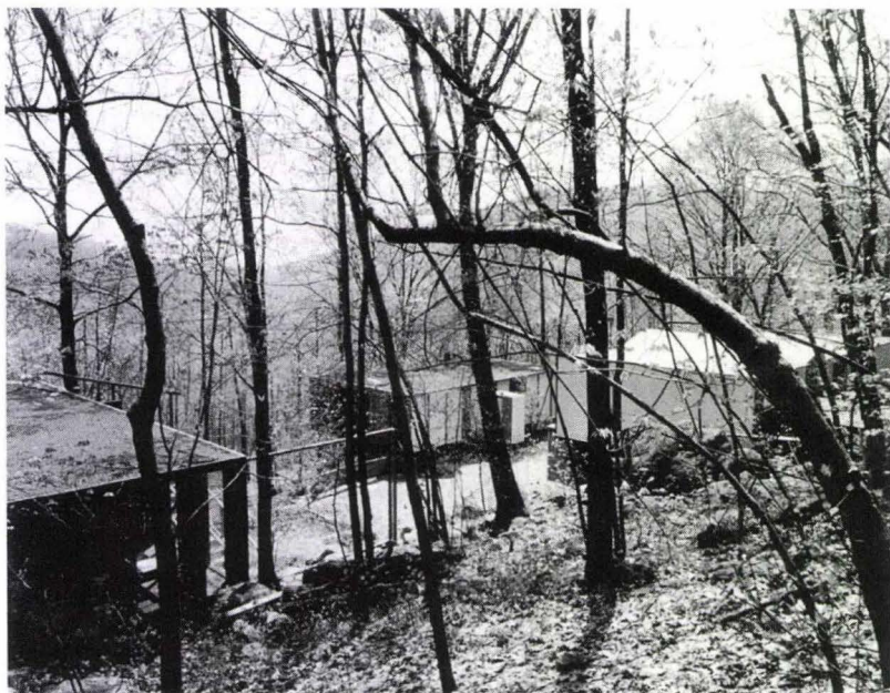
Figure 5.1 Paul Williams, Gatehill Cooperative Community, upper square, c. 1956. Western facade of Williams-Cage House at lower left.
