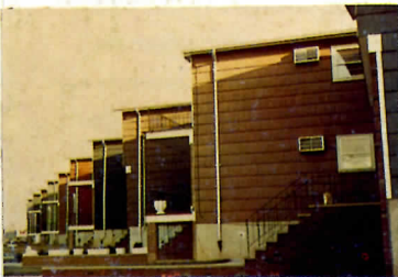
Housing Development, front view, Bayonne, New Jersey
