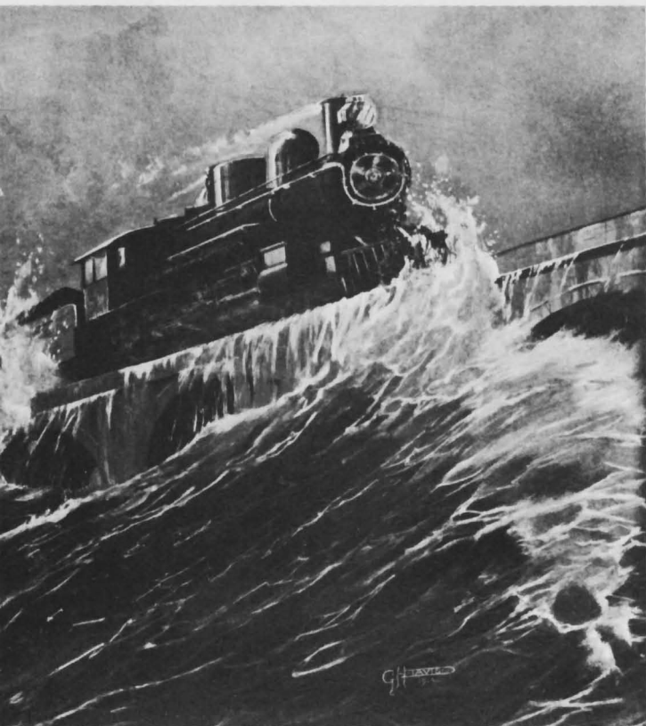
CUBA—THE LINE SWEEPED BY STORM
