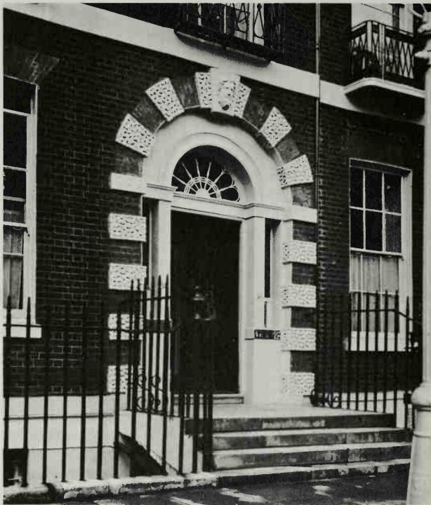
Doorway in Bedford Square, London. Black painted walls with white joints; stone castings around doorway; area wall, mouldings and reveals-painted in light color
