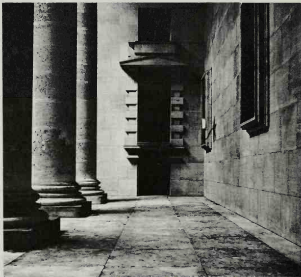
Police Headquarters, Copenhagen. Passageway in rectangular courtyard
