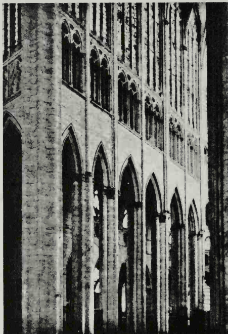
Chancel wall in Beauvais Cathedral. The bays are very tall and narrow and cannot be perceived singly but must be experienced as a continuous rhythm
