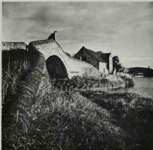
An English bridge of the great canal-building period at the beginning of the 19th century. Example of a "soft" form made of brick
