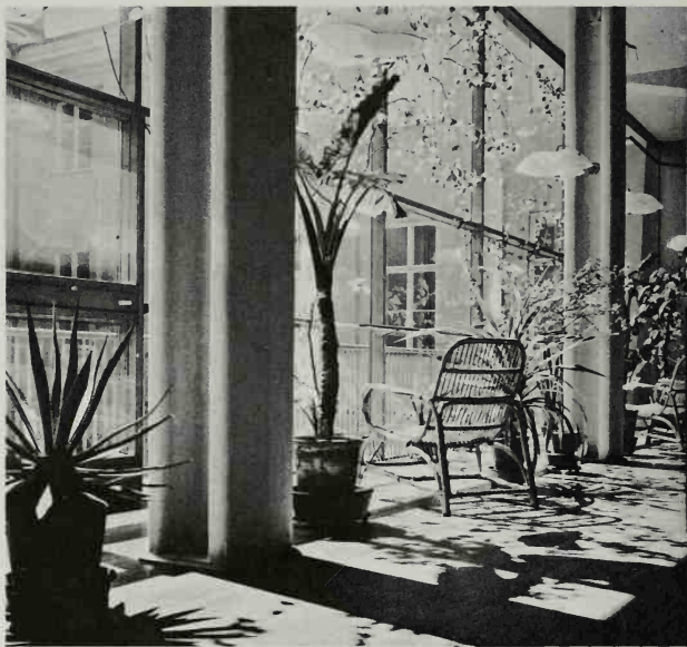
E. G. Asplund: City hall in Gothenburg, Sweden. The large window facing outer court. To avoid harsh shadows the steel shafts were covered and given soft contours
