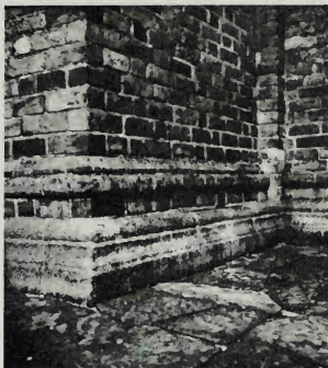
Medieval masonry, Roskilde Cathedral, Denmark
