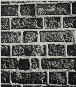
Medieval masonry of large bricks
