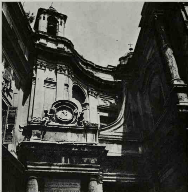
Detail of S. Maria della Pace, Rome, seen from point C on plan p. 69
