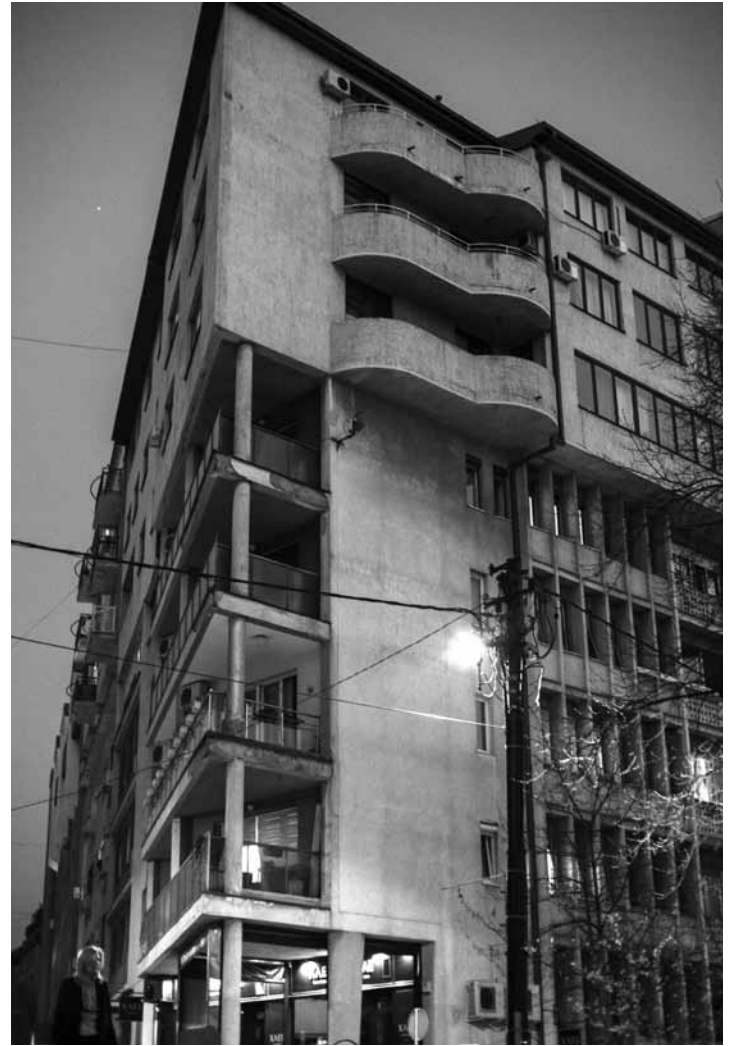
As time progressed, roof extensions in Belgrade grew both in size and ambition.
