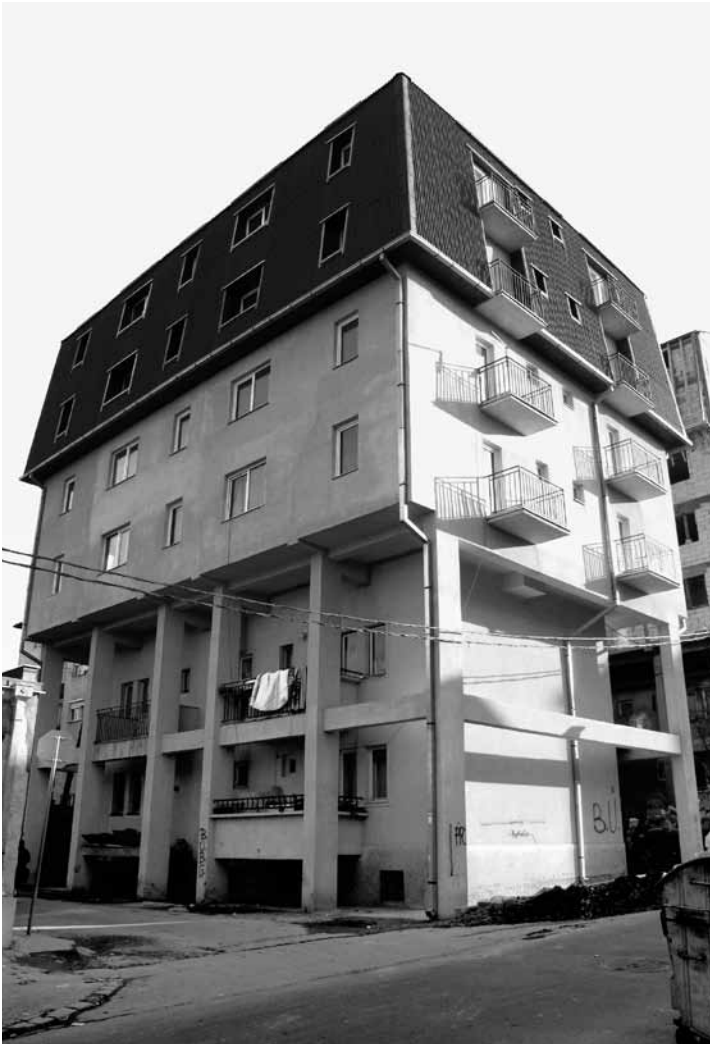
A typical extension of a Russian Pavilion, expanding its floor space as far as possible over the existing structure, thus enhancing the effect of a house sitting on top of another house. In the background, a glimpse of another extension in progress (photo taken in 2004).
