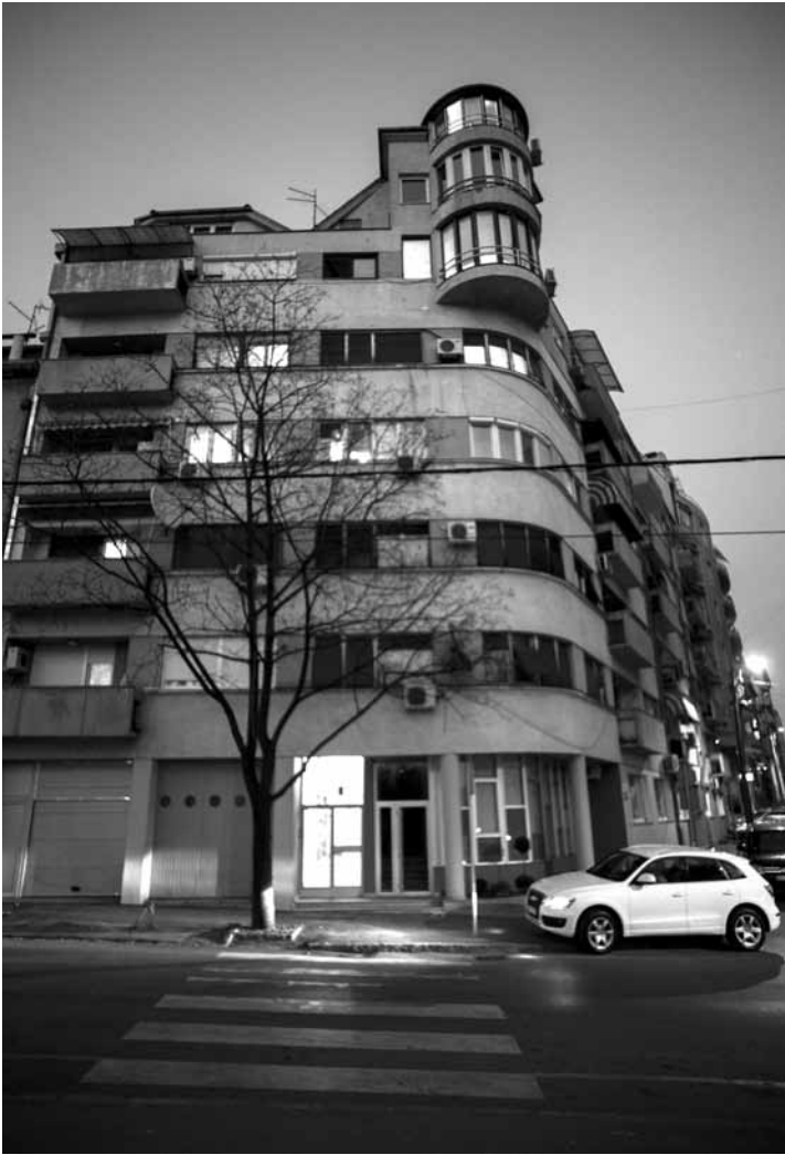
This building from the 1960s was originally designed as a single unit with two separate entrances, for two owner-councils. This enabled two different investors to build two different extensions on the same building.
