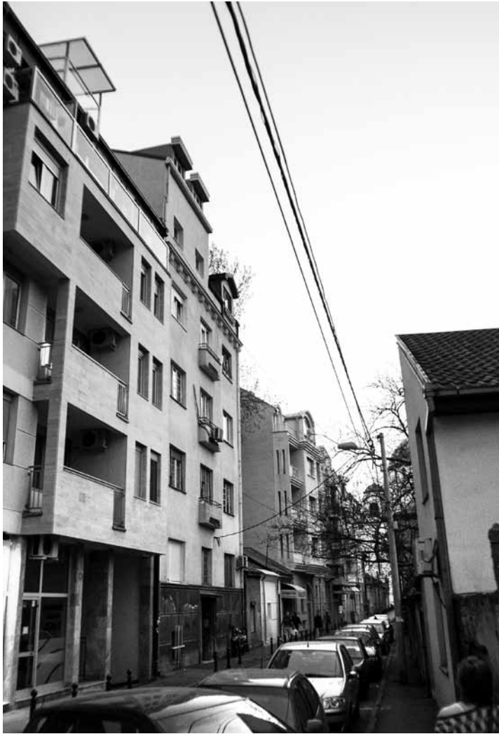
Most of the newly constructed buildings have extra-legal spaces embedded in them. The space below the roof and parts of the last floor are built as apartments and sold on the market, despite being designated as common storage areas in the construction permit.
