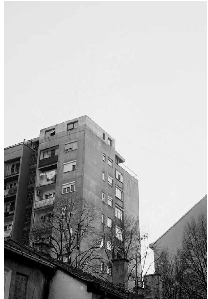
A small-scale, single apartment roof extension on the top-right corner of a 1960s high-rise.
