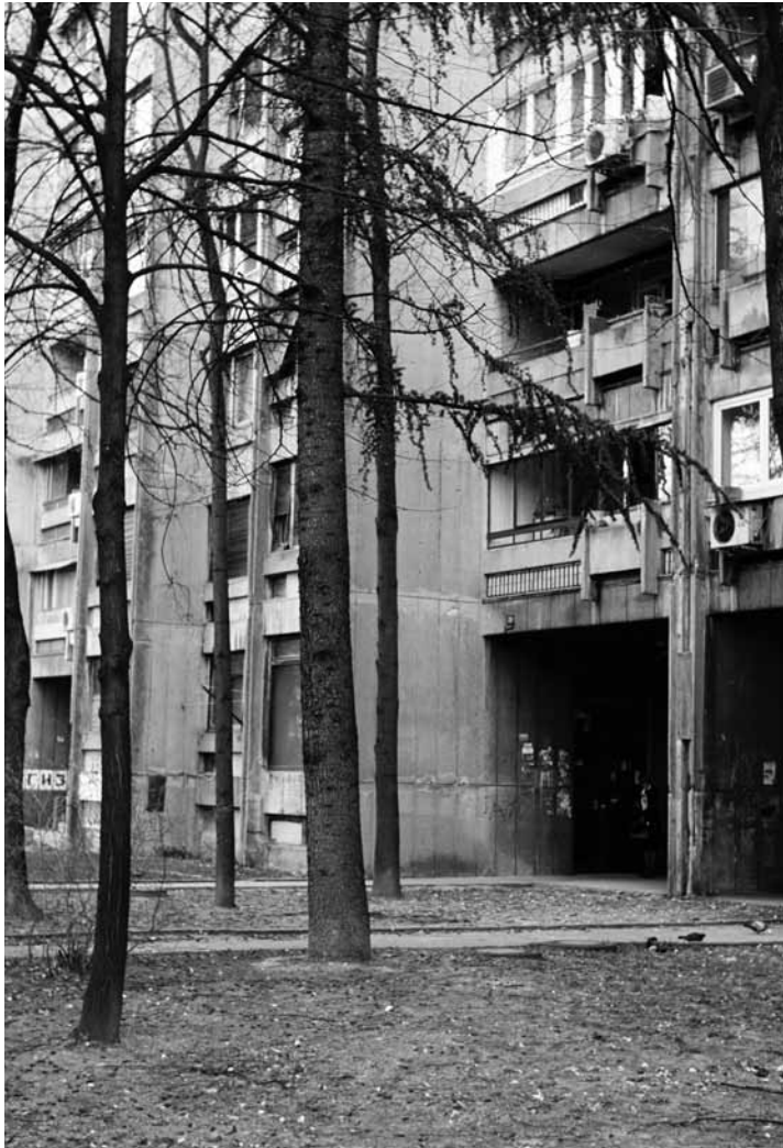
Following the housing privatization, new owners started making small modifications to their industrially produced apartments in order to suit their needs. The most common modifications were the expansion of living space to the balcony area, and the addition of visible, external air conditioning units, as seen here.
