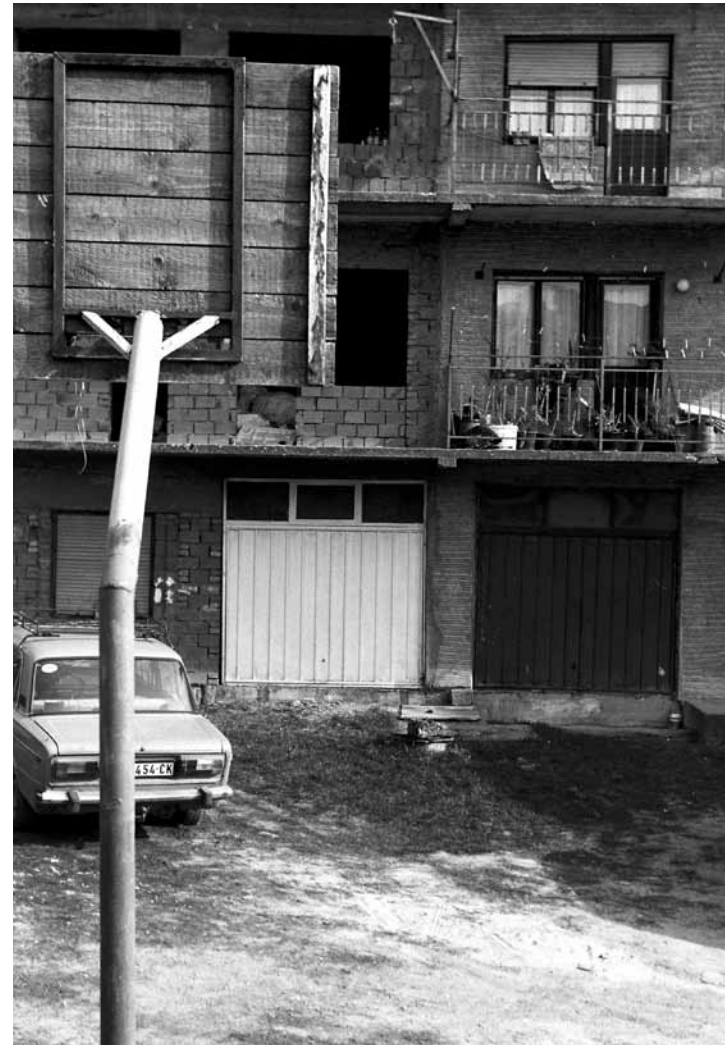
A self-built duplex for two brothers and their families in Kaluderica; both floors in various stages of completeness. Due to the lack of proper public space, the front garden became a playground for the local community.
