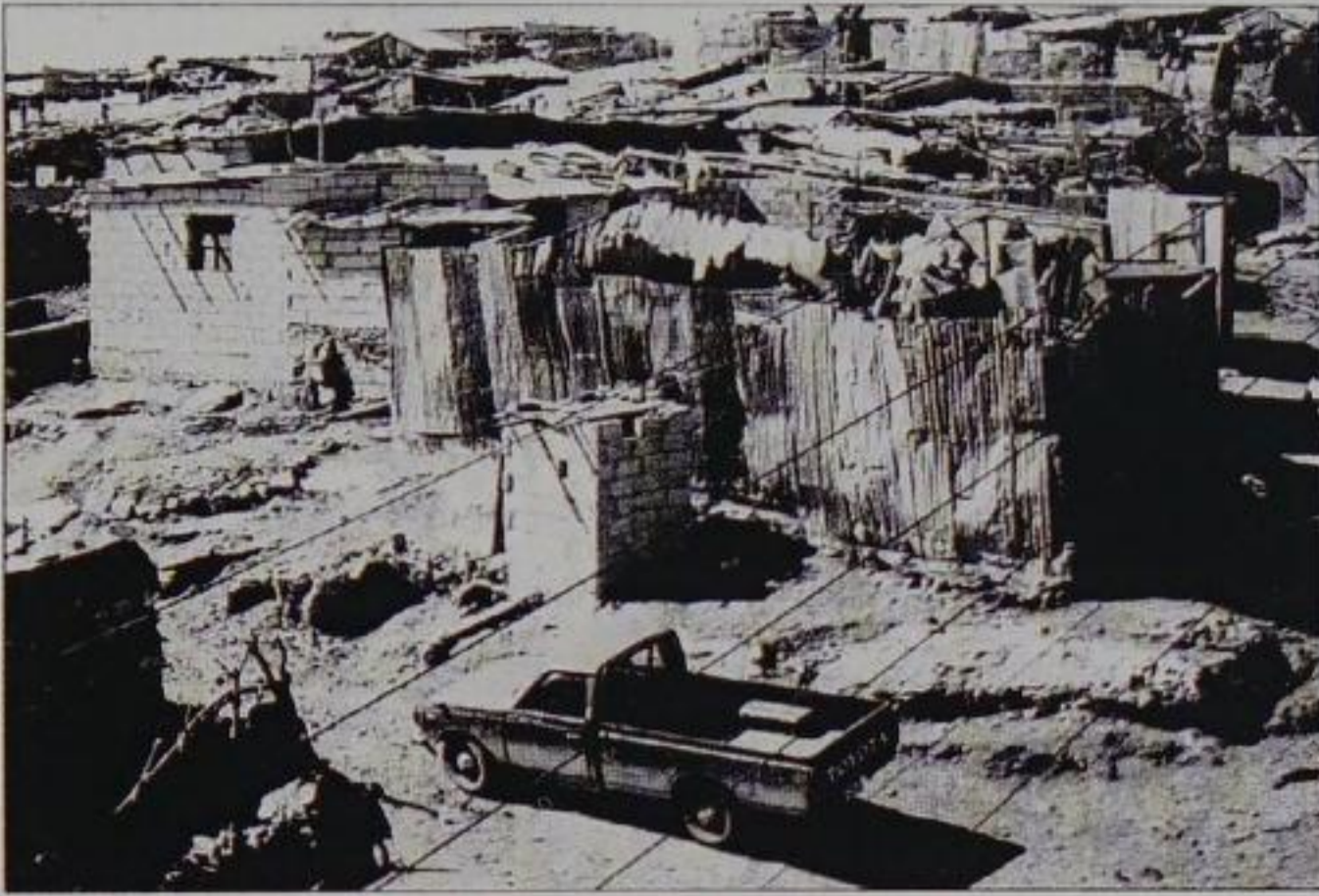
Ramshackle sheds in East Wahdat before the upgrading programme
