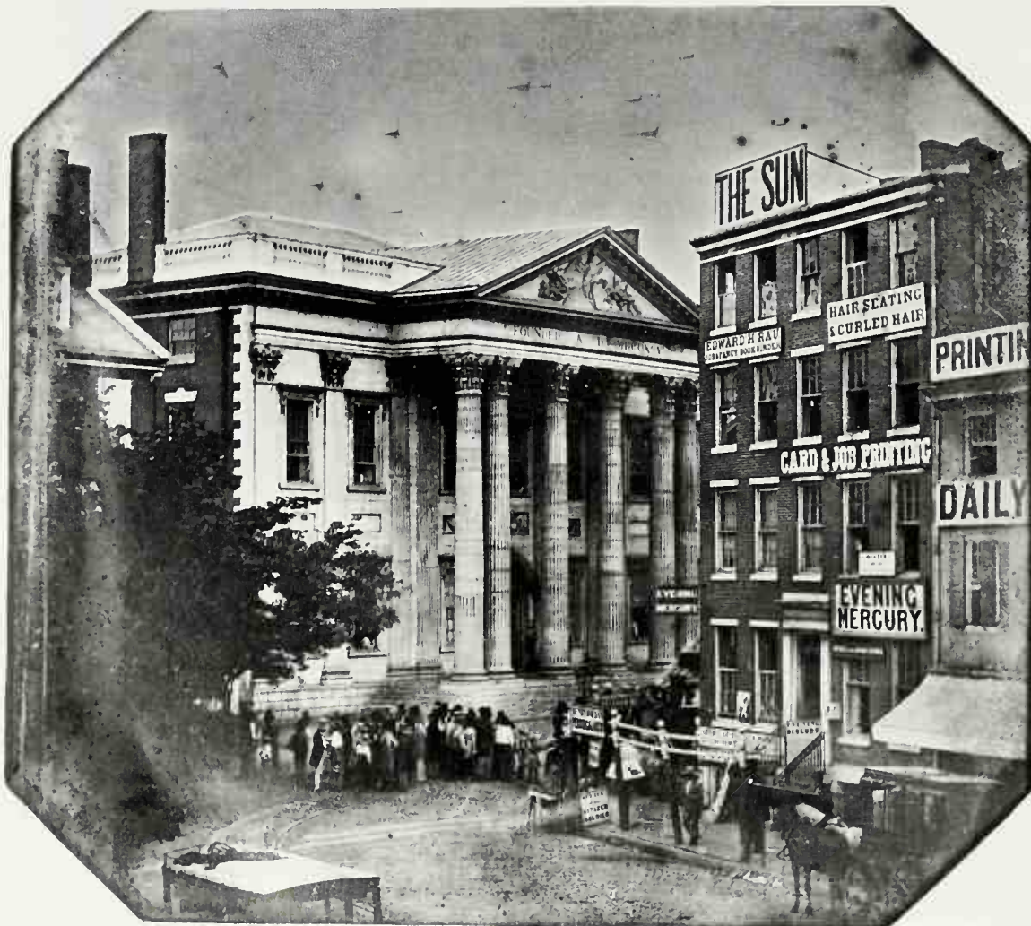
16. WILLIAM and FREDERICK LANGENHEIM. Girard Bank, May, 1844. Daguerreotype. Library Company of Philadelphia.
