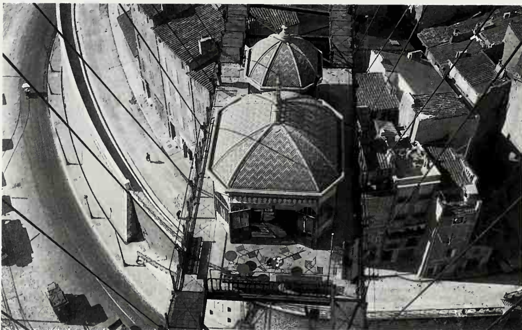
505. HERBERT BAYER. Pont Transbordeur, over Marseilles , 1928. Gelatin silver print. © Estate of Herbert Bayer.
