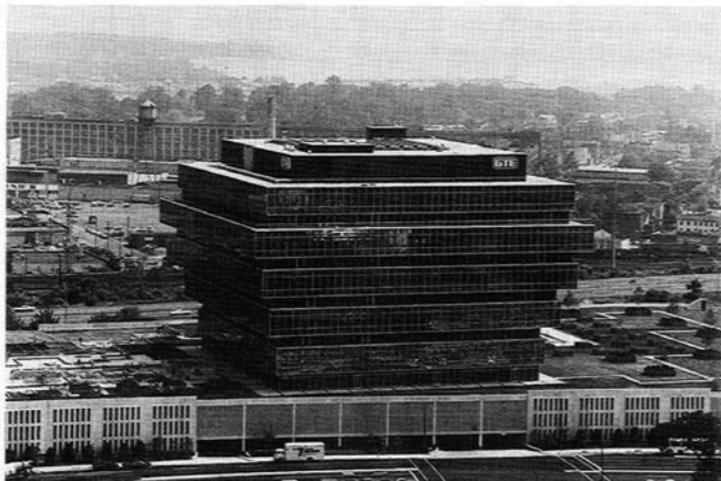
Owner and general contractor: F. D. Rich Company, Inc.; architect: Victor H. Bisharat, AIA; structural engineer: Werner Jensen of Werner Jensen and Adams; fabricator and erector: New England Iron Works
