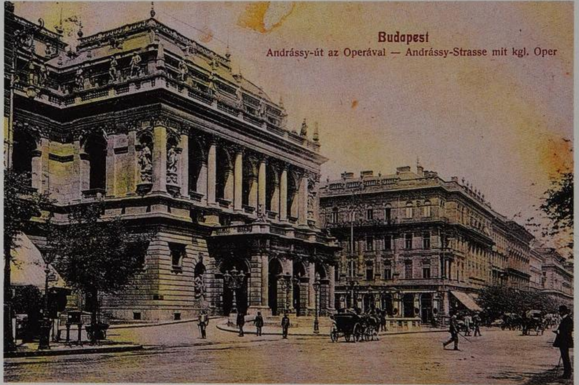
Opera house on Andrassy Avenue, Budapest, 1910s
