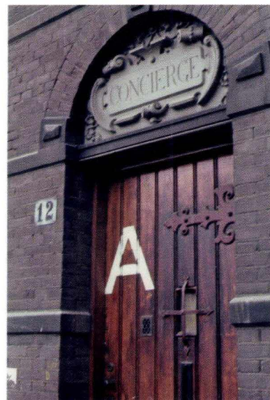
The squatted caretaker's house, part of a former prison complex at the Kleine-Gartmanplantsoen 12, Amsterdam, 1979.
