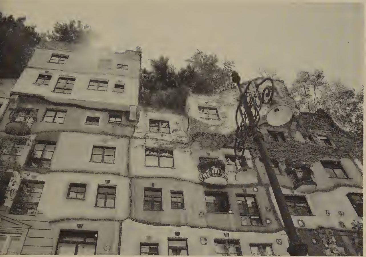
Friedensreich Hundertwasser, idea and concept | Architect and original coauthor: em.o. Univ.-Professor DI J.Krawina | Architect and planning: DI Peter Pelikan, architect | Hundertwasser House, Vienna | 1985
