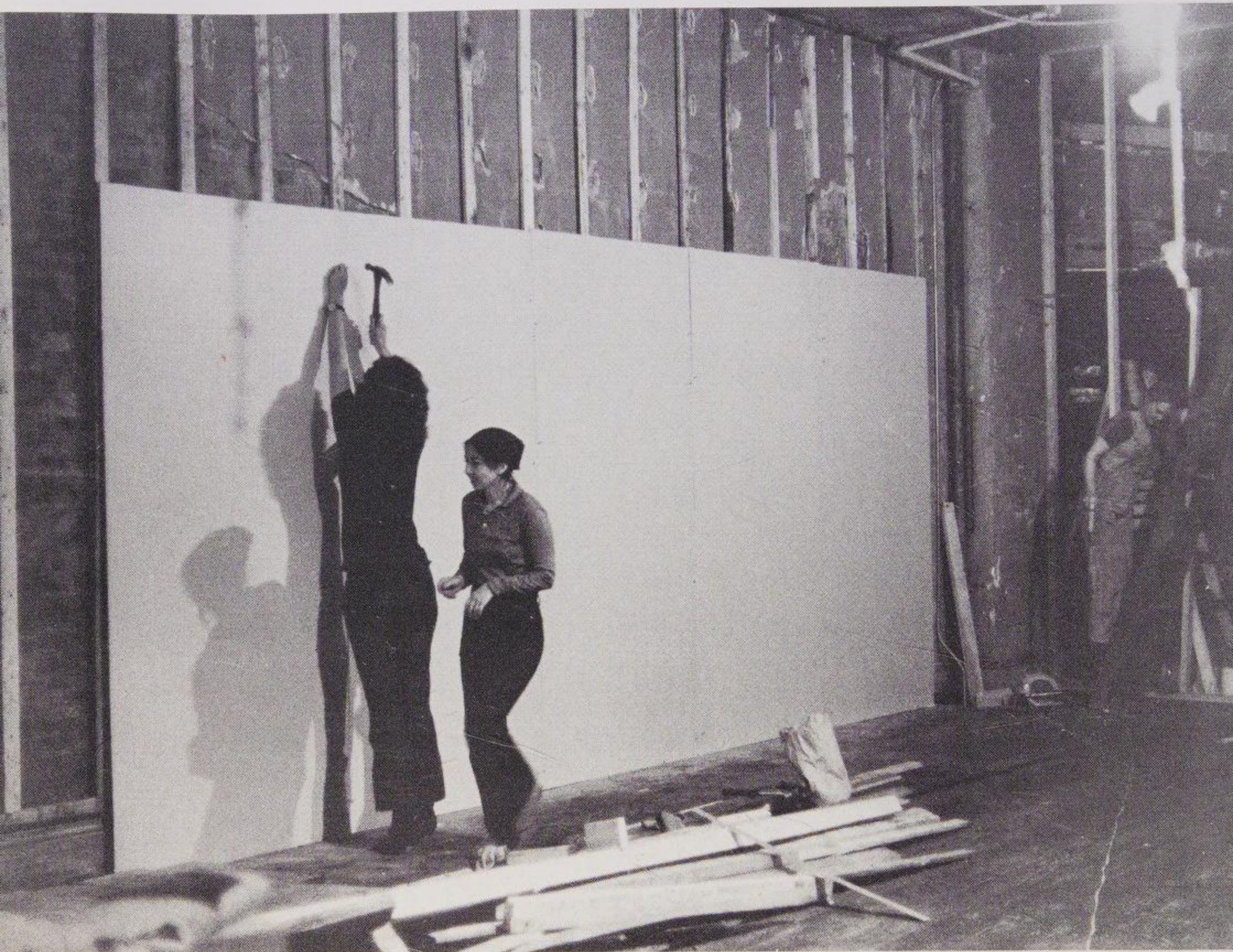
A.I.R. members hanging wallboard at A.I.R., 1972. Courtesy of A.I.R. Gallery. Photograph by David Attie.
