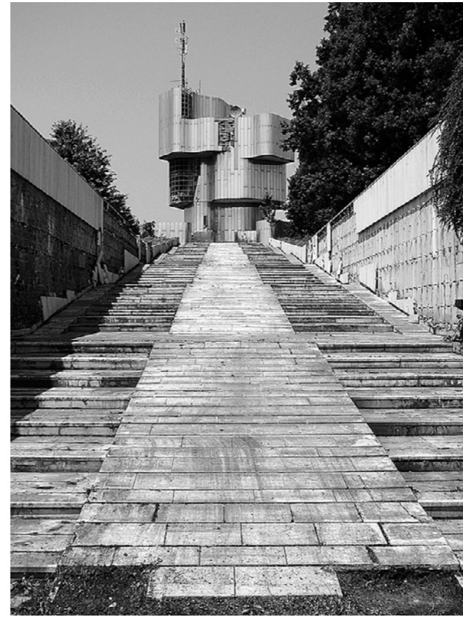
▲ Vojin Bakić, Petrova Gora (finished 1981), present condition
