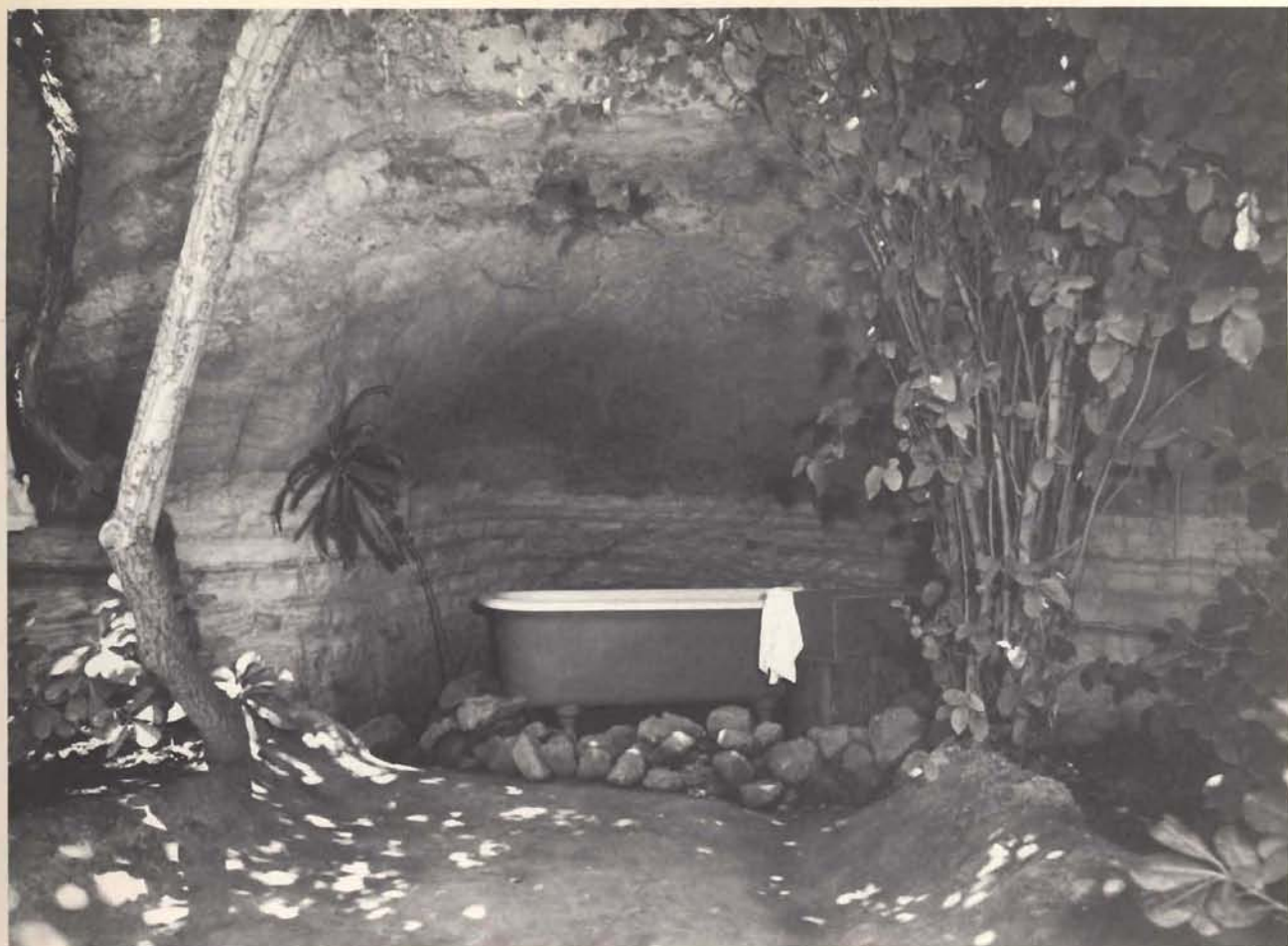
AS YOU COME ACROSS THE BRIDGE OVER THE POND ON THE FAR SIDE, YOU SEE A BATHTUB. THIS WAS BALDASARE'S BATHROOM. THE TUB SITS UPON BOARDS. UNDER THE BOARDS IS A HOLE THAT THE BATH WATER DRAINED INTO. ABOVE GROUND, OVERHEAD, HE HAD A METAL TANK TO HOLD THE WATER. HE HAD A HOSE ATTACHED TO THE TANK COMING DOWN TO THE BATHTUB. IN FRONT OF THE ALCOVE HE HAD A PIECE OF CANVAS. OF COURSE, LIVING ALONE MOST OF THE TIME, HE PROBABLY DIDN'T NEED IT.
