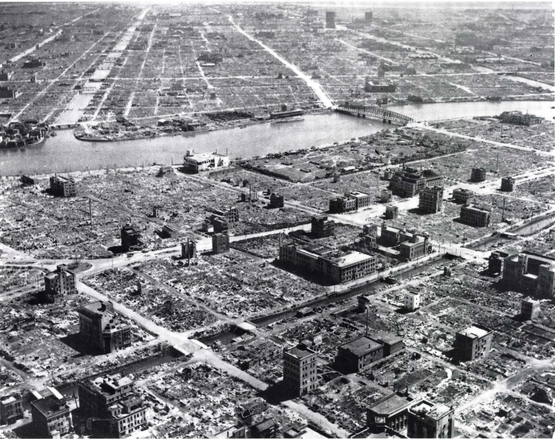
FIGURE 3.1 DOWNTOWN TOKYO AFTER THE FIREBOMBING OF MARCH 10, 1945
