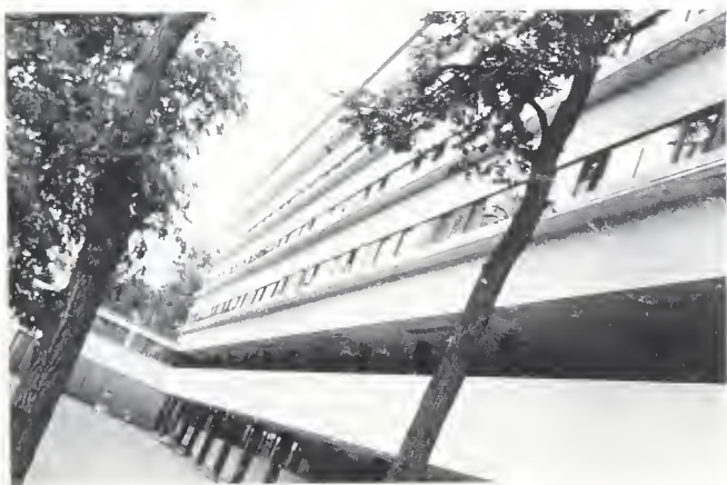
Above and right: the Narkomfin building designed by Ginzburg, 1932. Leica.
