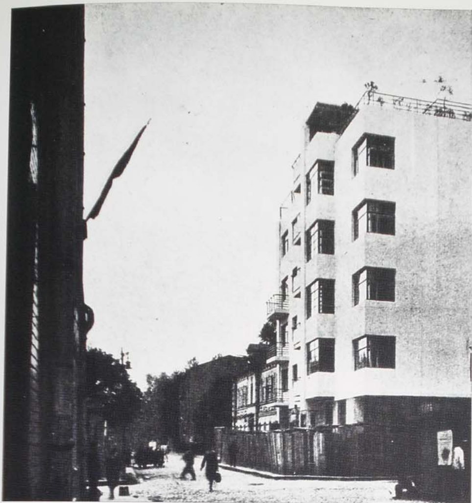
a: Moisei Ginzburg. Apartment and communal housing block for the State Insurance Bureau, Gostrakh, built 1926-27: street view.
