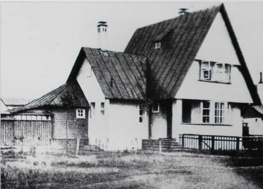
a: Nikolai Markovnikov, proposal for a two-storeyed terrace of semi-collectivised workers' housing with communal dining room, 1925: ground and first-floor plans. b, c: Housing type 60 in timber, for Sokol Garden Settlement, Moscow, 1925-26: photograph soon after completion, ground-floor plan. d: Housing type 58 in the Gerard blockwork system, for Sokol Garden Settlement, Moscow, 1926: photograph soon after completion. e: Proposal for a two-storeyed 'Communal house of economic type' compared with the high-rise 'Communal house of the favourite economic type - a model which is without economic foundations and therefore represents an impractical architectural fantasy', 1928.
