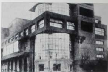
Ilya Golosov, Zuev Workers' Club, Moscow, 1927-29: corner detail, photograph 1989.
