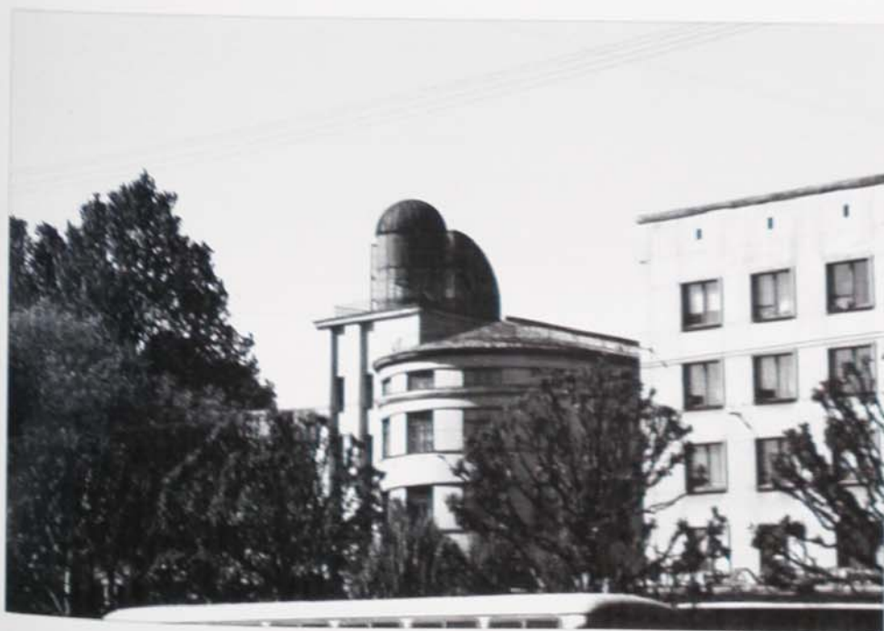
f: Secondary School named for the Tenth Anniversary of the Revolution, Leningrad, 1927; detail of teaching block and observatory.
