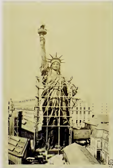
fig. 7. Albert Fernique. Frédéric Auguste Bertholdi's Statue of Liberty, under construction at the Gayet-Gauthier foundry, Paris. 1884. Albumen print, 7 1/16 x 5 1/16" (20.2 x 12.9 cm). Musée Carnavalet, Paris
