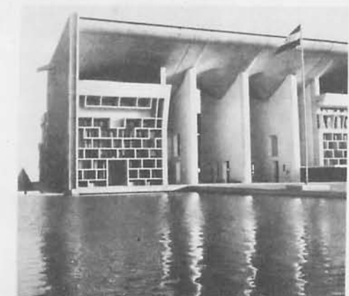
132. High Court building, Chandigarh, 1951-1956; Le Corbusier
