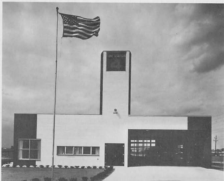
116. Fire Station No. 4, Columbus, Indiana, 1965-1967; Venturi and Rauch
