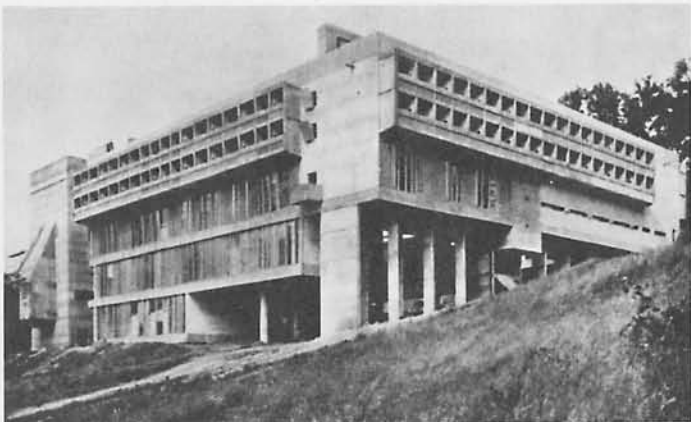
133. Monastery of La Tourette, Evreux, France, 1956-1960; Le Corbusier
