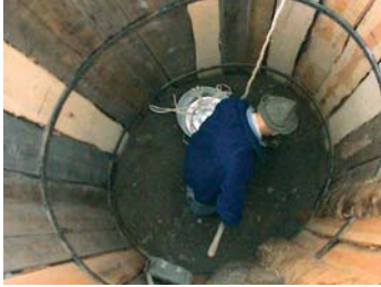
During the installation work
