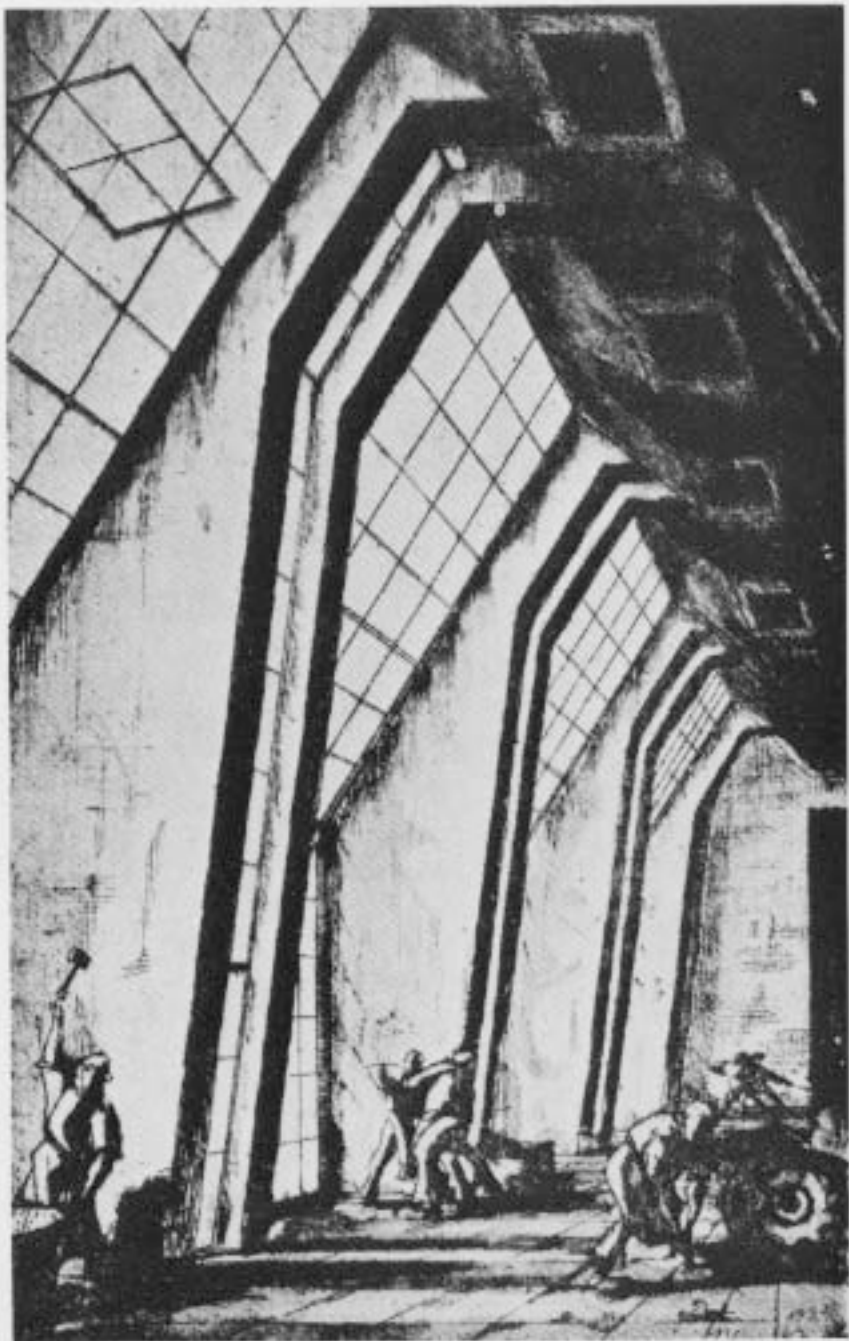
9 E. I. Norvert. New boiler room for an electrical power station outside Moscow.
