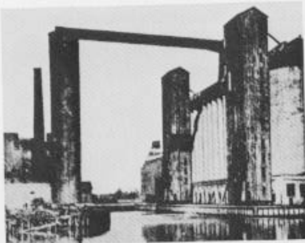
Elevator in Buffalo
