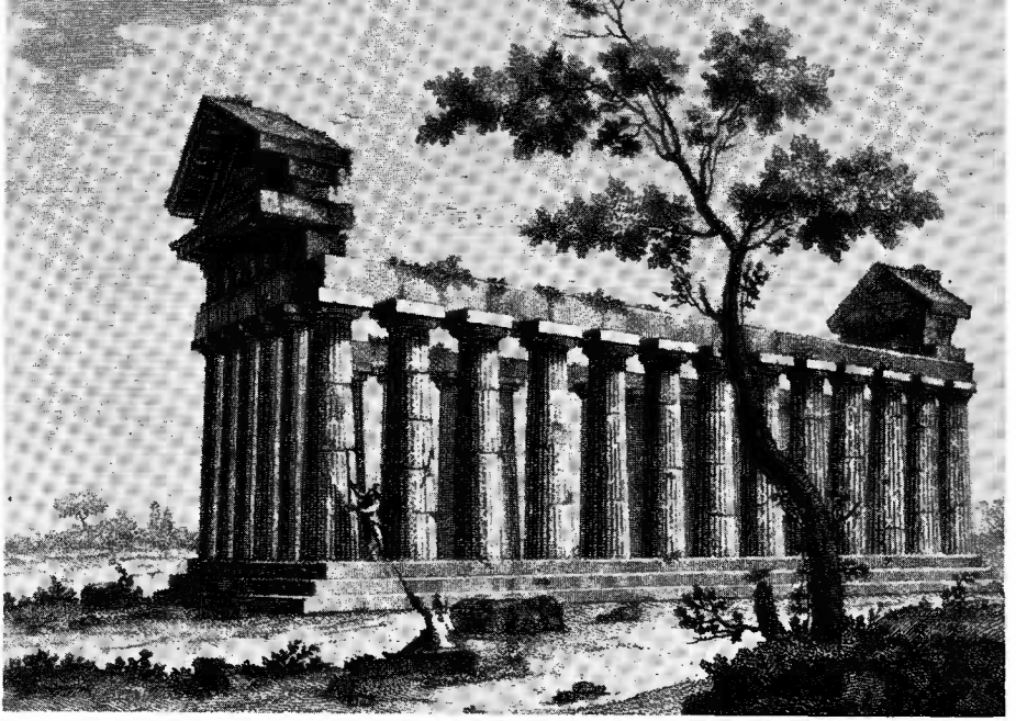
3. Temple of Concord, Agrigento . Engraving from the Italian edition of 1783–4 of Winckelmann, Geschichte der Kunst des Alterthums and other essays. One of the few works of classical architecture about which Winckelmann wrote.
