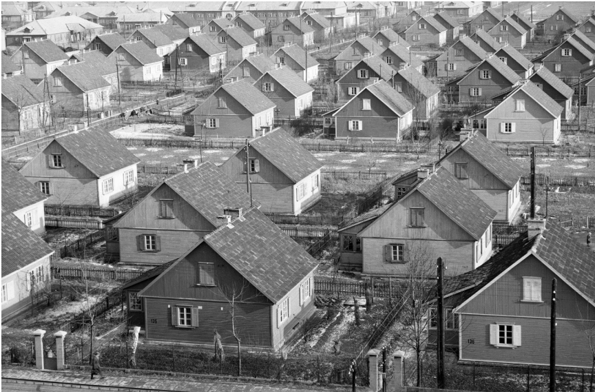
Figure 2.2. The wooden houses built for Soviet workers in Jelonki, a suburb of Warsaw. Subsequently renamed the Przyjaźń (Friendship) housing estate and used until today, partly as student and faculty housing for the University of Warsaw. Photograph courtesy of the National Digital Archive.
