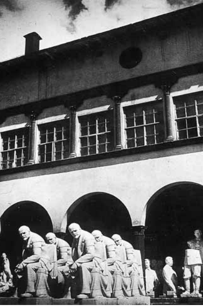
2.36 Courtyard of the Sculpture House in the Vsekokhudozhnik Commune, Moscow (architect: Georgii Golts), for the mass reproduction of Lenin statues, anonymous (unofficial) photograph, 1932–1936.
