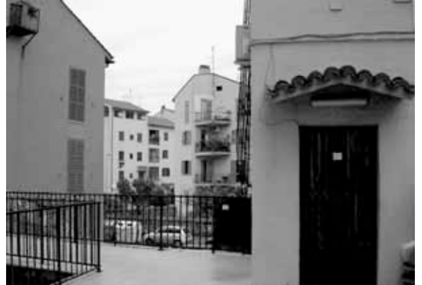
Fig. 4 The casual front entrances along the raised walkway were intended to produce more intimate thresholds between public, semi-public, and private domestic spaces. The scale and detailing of the door stoops and awnings mimic the vernacular character and ambience of an Italian village. It was imagined that the design would better suit the future inhabitants of the state-sponsored housing project.
