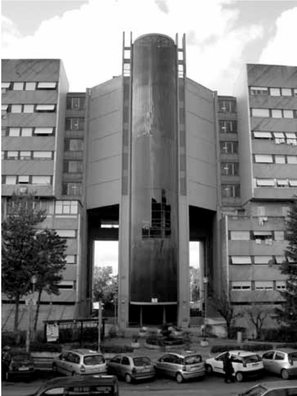
Fig.3 The elevators frequently malfunctioned and, along with the entryways, were often targeted by vandals. By late 1983, nearly 700 families were illegally occupying the building. The squatters settled into the fourth floor of the main building, which had originally been designed to support boutiques for artisan products, offices and commercial activities. This design strategy emulated the modern housing typology of the Unité d'Habitation, designed by Le Corbusier in the early 1950s.
