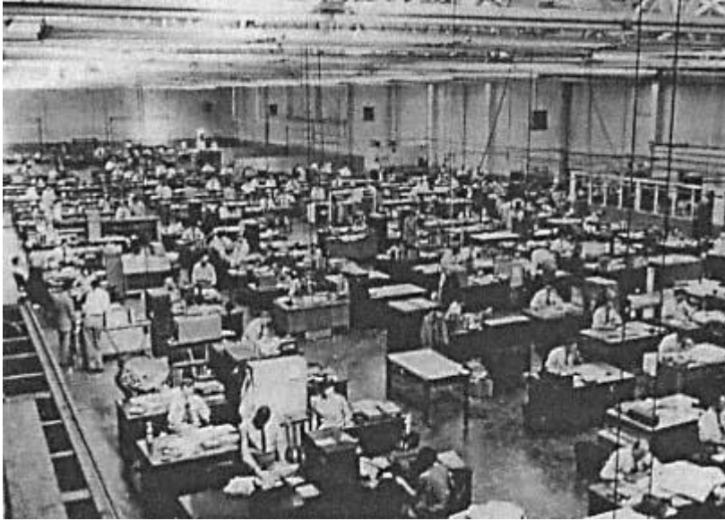
Figure 1 "Computing" at North American Aviation, Los Angeles, California, ca. 1952. It was this room, and the flow of information that went through it, that was replicated by the architecture of the stored program digital computer. Photo credit: National Air and Space Museum
