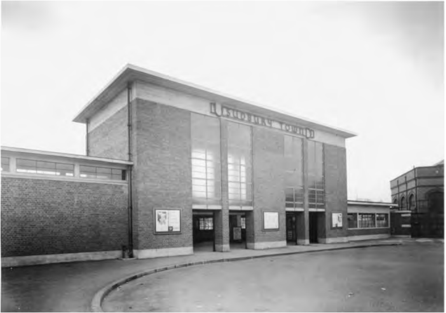
FIGURE 5.10. Sudbury Town station after being rebuilt, 1934. Reproduced by permission of the London Transport Museum.
