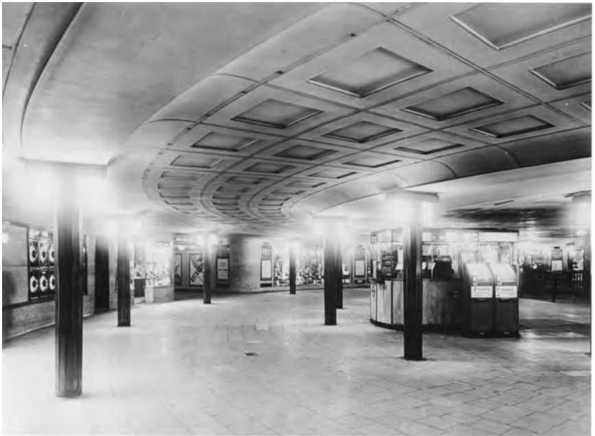
FIGURE 5.5. Piccadilly Station booking hall after renovation—"a scene that would make a perfect setting for the finale, or indeed, the opening chorus of an opera." Reproduced by permission of the London Transport Museum.
