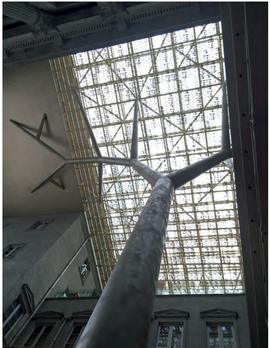
Interior of the National Gallery Singapore, detail of the tree structure, 2015 (photograph by the author)
