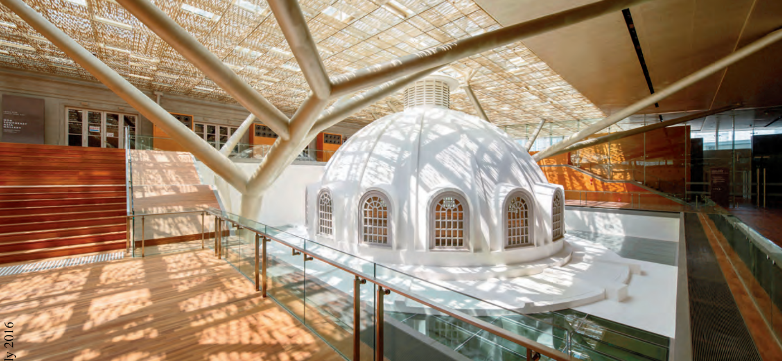
Level 4M of the Supreme Court Wing, National Gallery Singapore, formerly the Supreme Court Terrace (photograph © Darren Soh)
