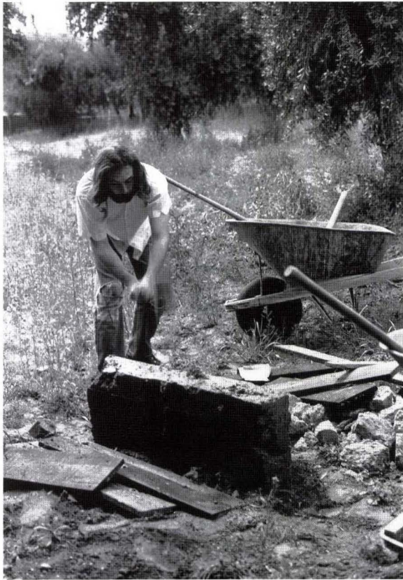
PARTICIPANTS BUILDING FORMS AND MIXING CONCRETE (TOP) AND BREAKING UP A CONCRETE FOOTING (BOTTOM) DURING TRACTS , BURBANK, CALIFORNIA, 1970 (PHOTOGRAPHERS UNKNOWN)
