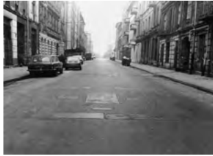
Construction in Process. Back in Łódź 1990, Micha Ullman's installation in the road surface on Wschodnia Street
