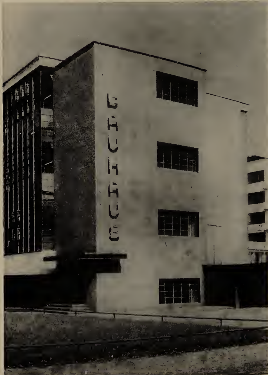
Figure 75. Walter Gropius, Bauhaus, Dessau, Germany (1925–26). Detail of exterior. Courtesy Foto Marburg/Art Resource, New York.
