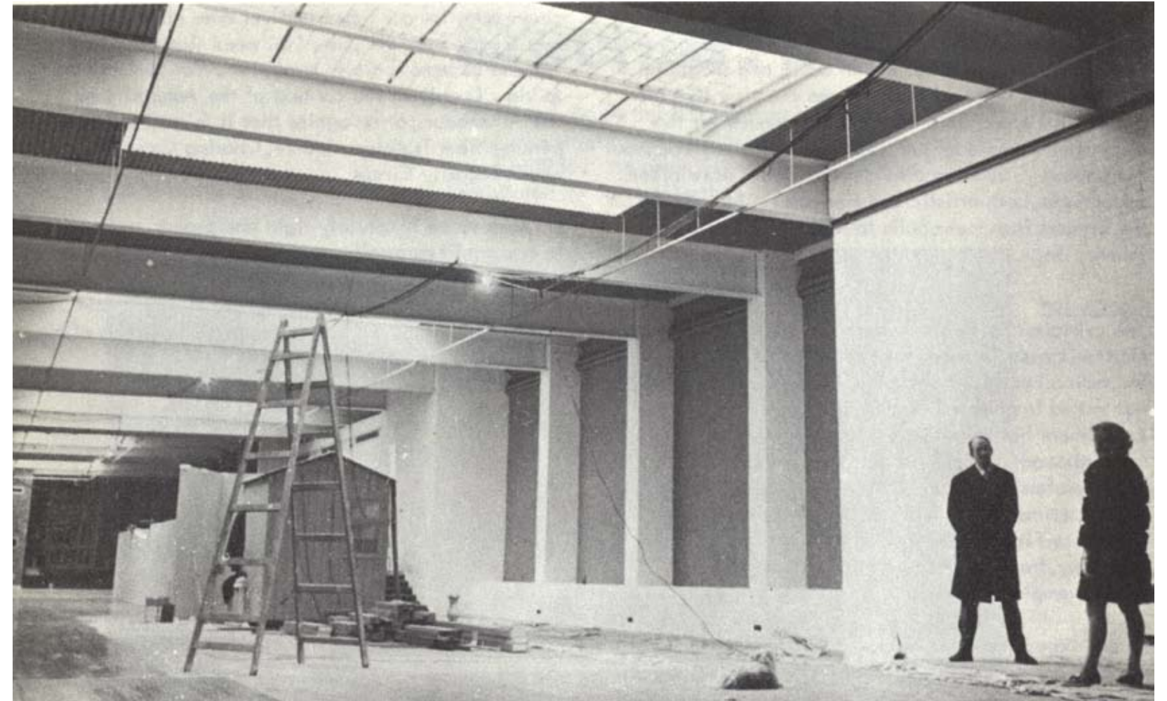
The ICA under construction, printed in the ICA Bulletin in 1968
