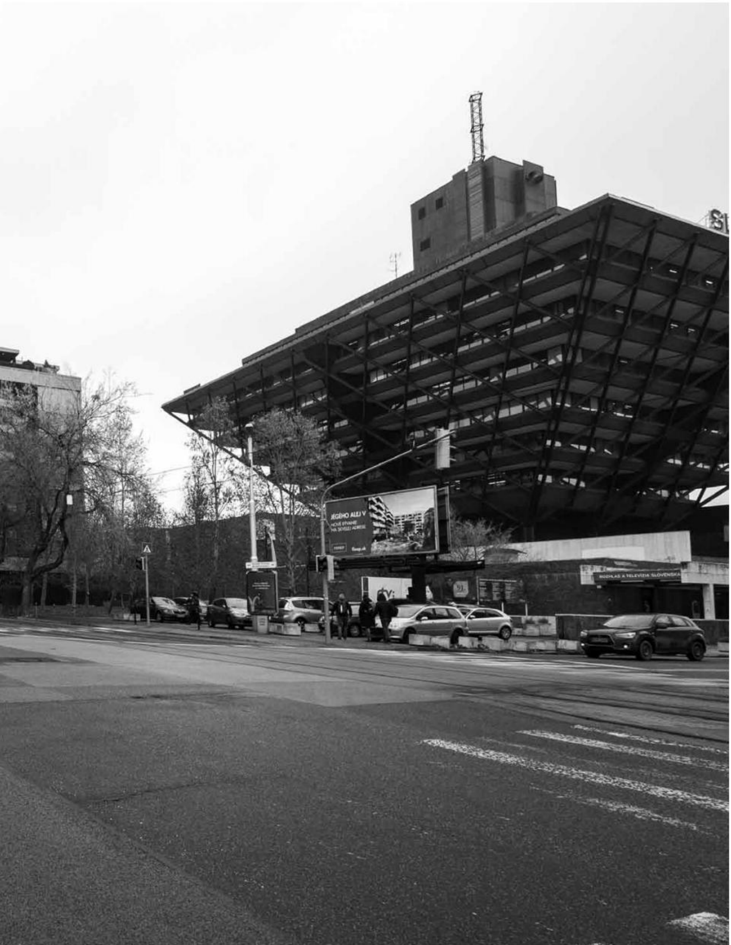
The space between the radio building and the former Postal Palace as the only realized fragment of the transverse axis vision, 2019 Photo: Olja Triaška Stefanovič
