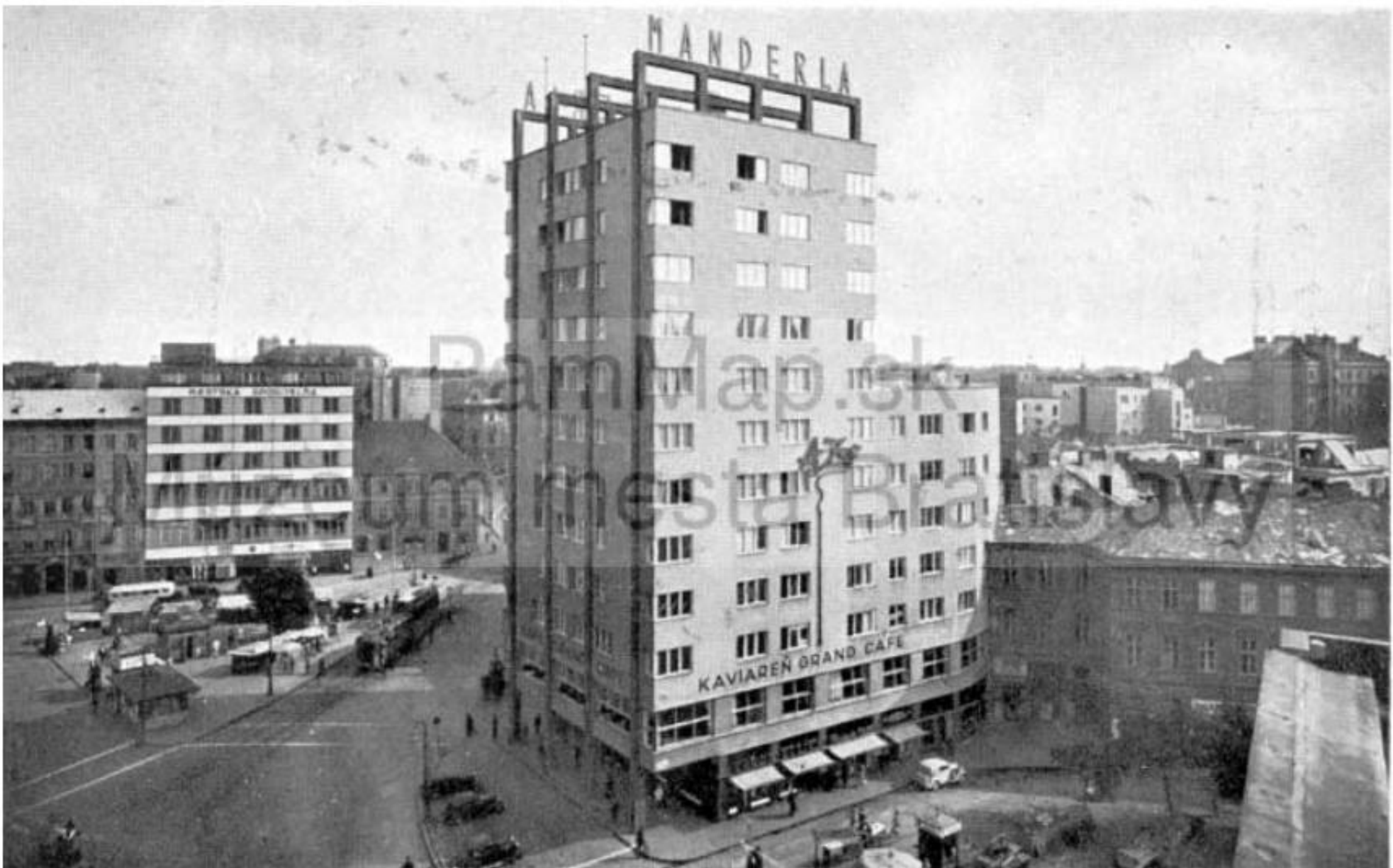
Lower part of today's Námestie SNP, around 1936, Manderla commercial and residential house in the foreground (Ch. Ludwig, A. Danielis, E. Spitzre, 1935) Source: Bratislava City Museum
