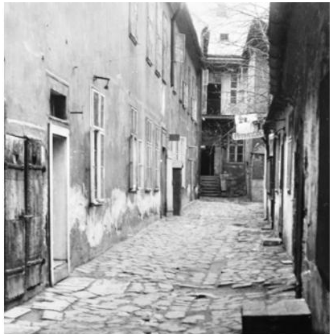
View of the yard before 1930 Source: Bratislava City Archives
