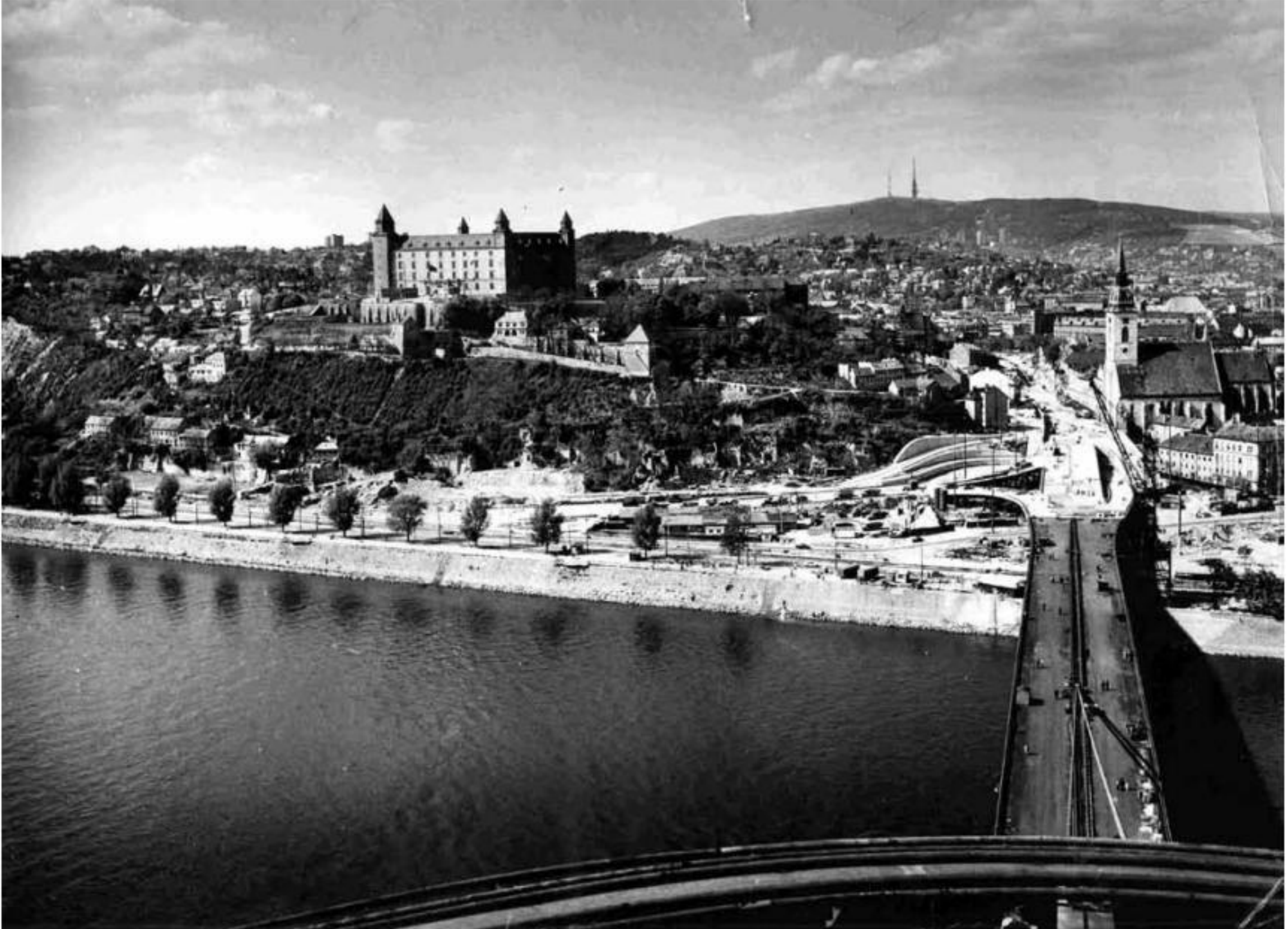
View of the construction of SNP Bridge and its connection to the inner city ring, around 1970 Source: Bratislava City Museum
