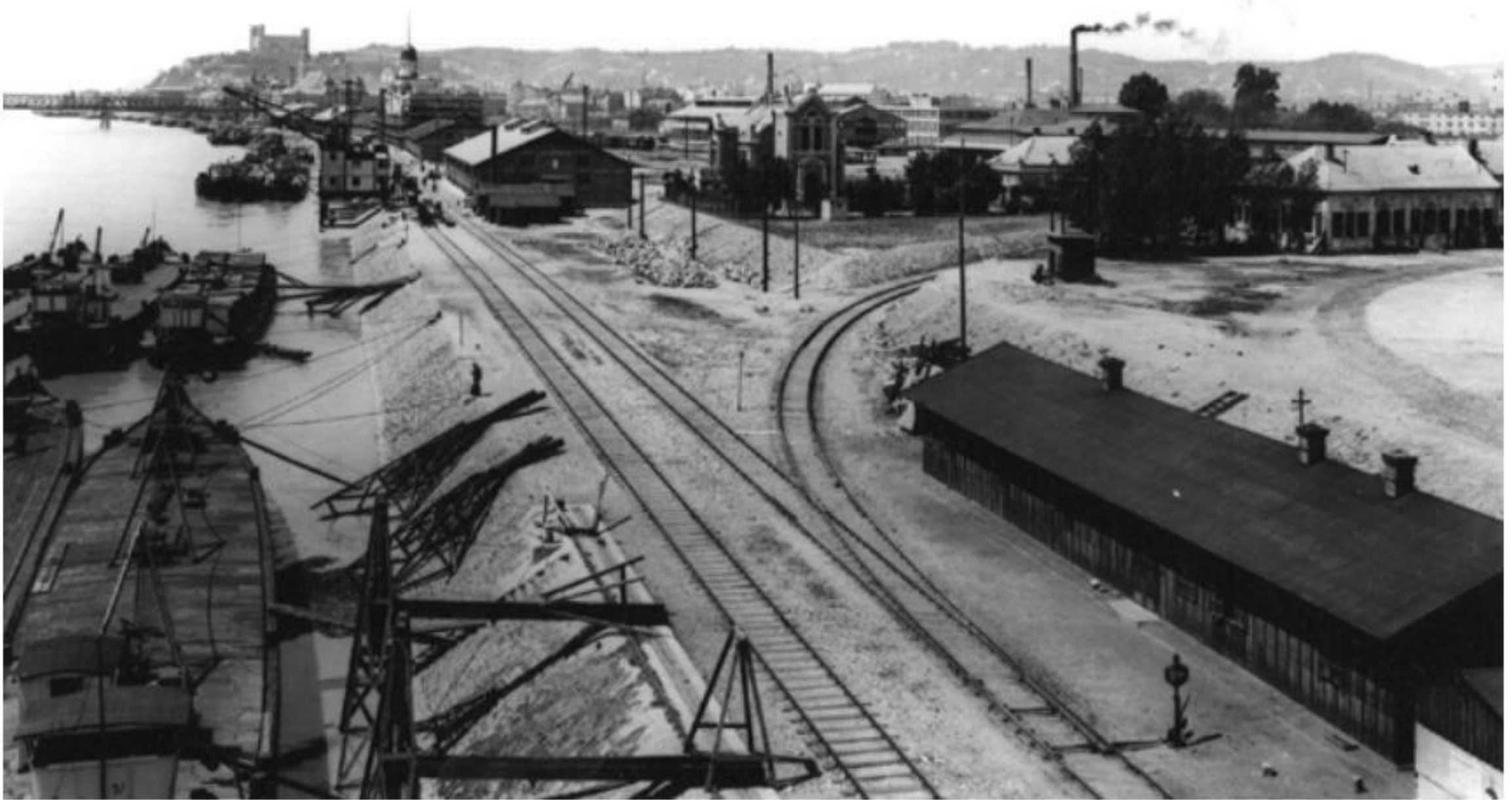
Danube river port around 1930 Source: The Monument Board of the Slovak republic archives
