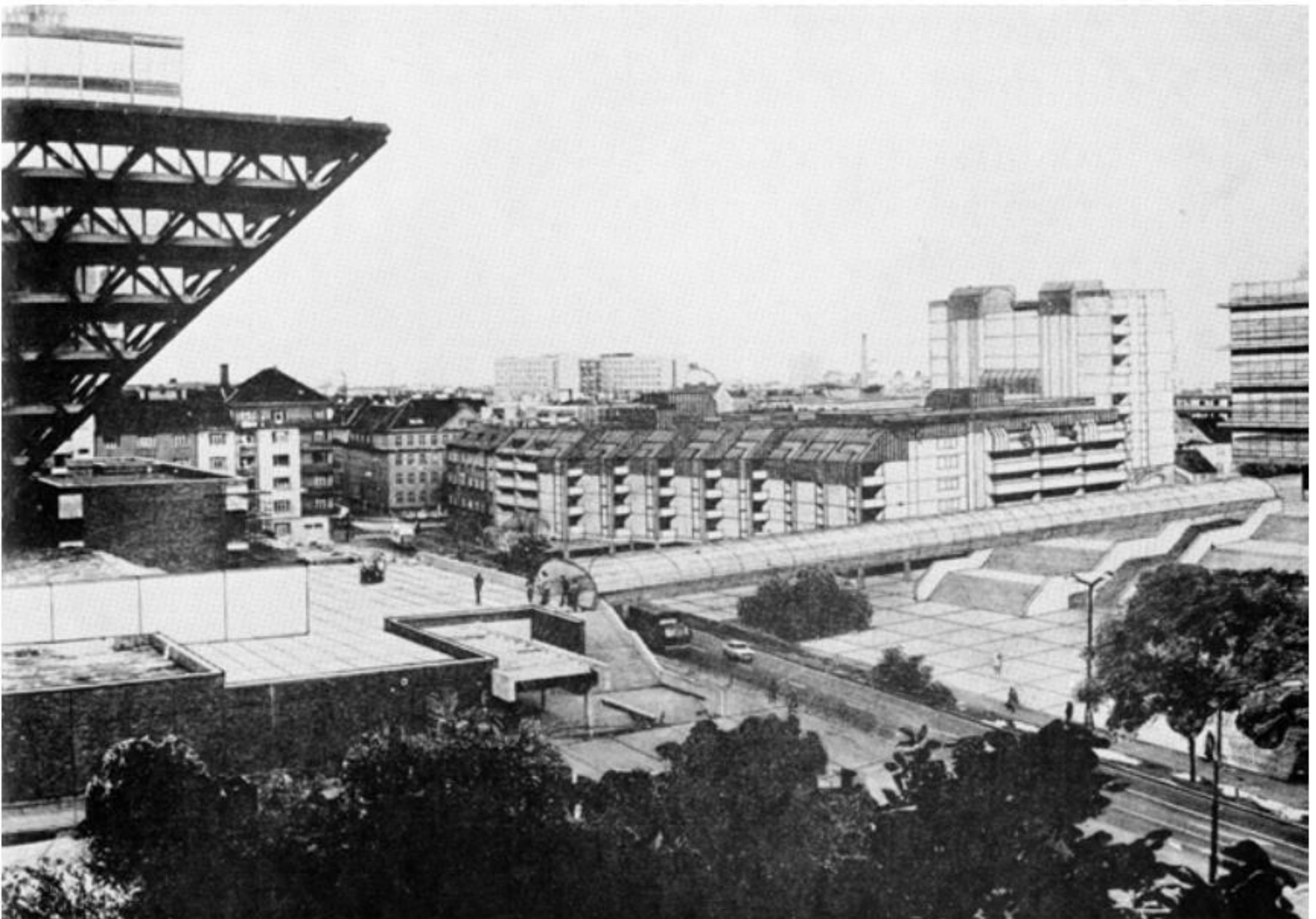
Starohorská mass housing, Štefan Svetko, Boris Džadoň, modified design using new panel technology, 1982 Source: Projekt, 1983
