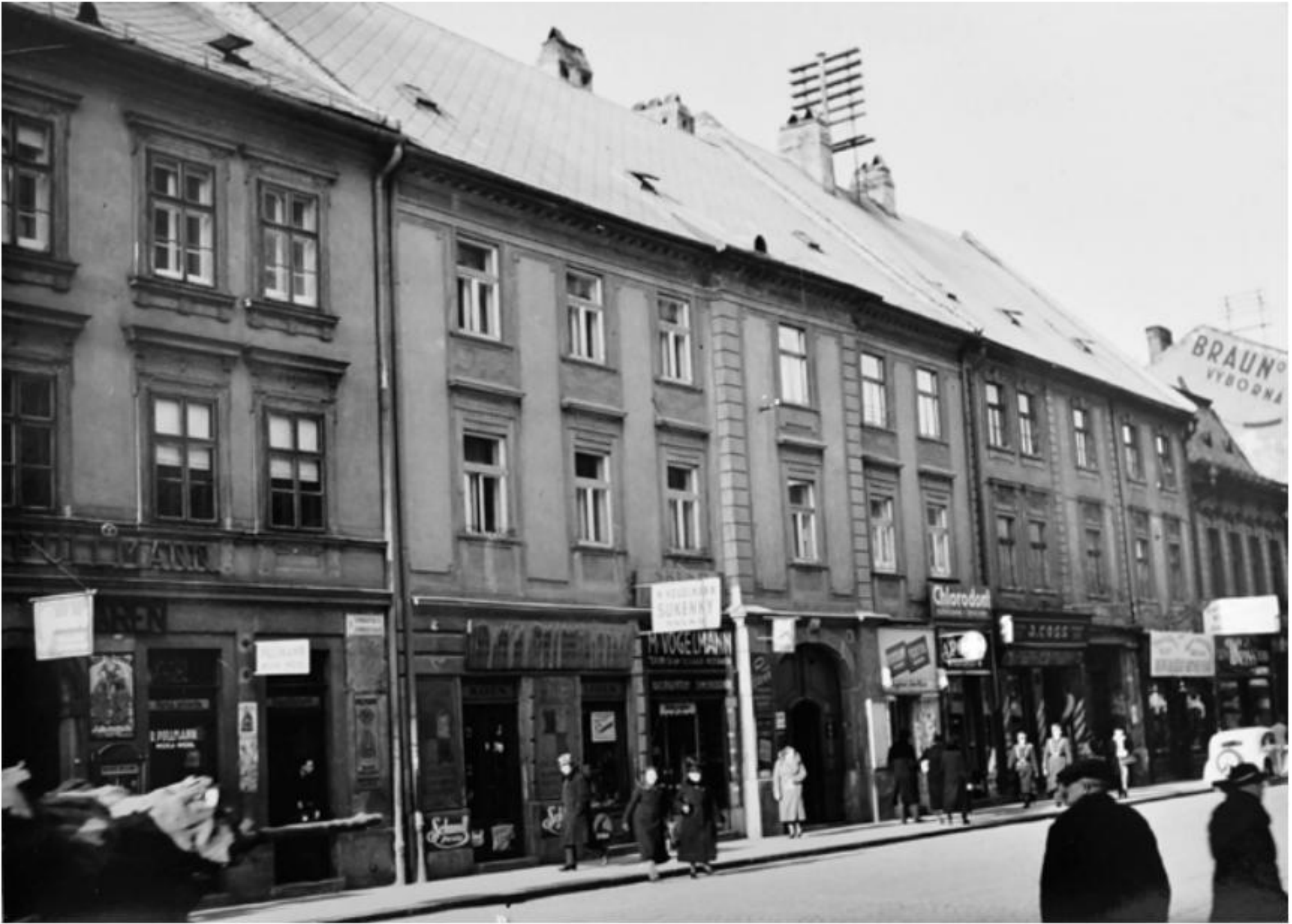
The House on Obchodná ulica No.23 before regulation Source: Bratislava City Archives
