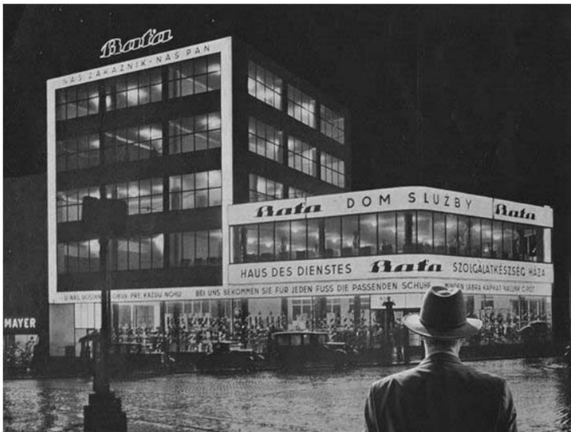
Bata House of Services, Hurbanovo námestie 6, V. Karfík, 1930 Source: Bratislava City Museum
