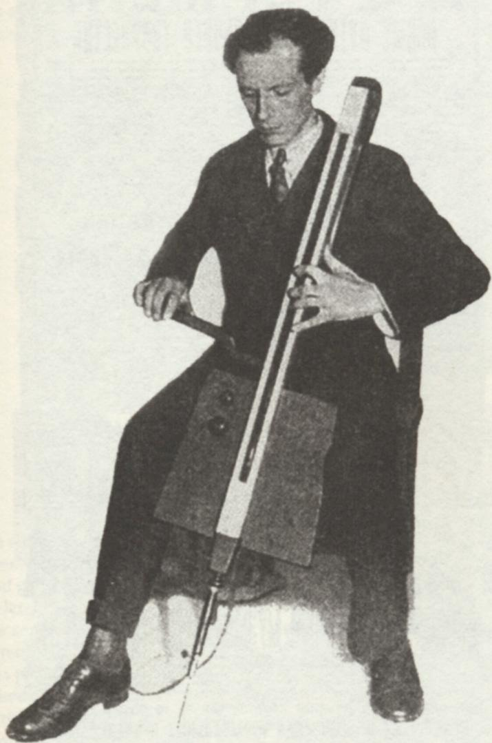
fig 2.4 Theremin demonstrating one of his fingerboard models. The position of the left hand on the neck defines the pitch of a sound while loudness is adjusted by the special lever reminiscent of a bow. *Popular Science Monthly*, 1932.
