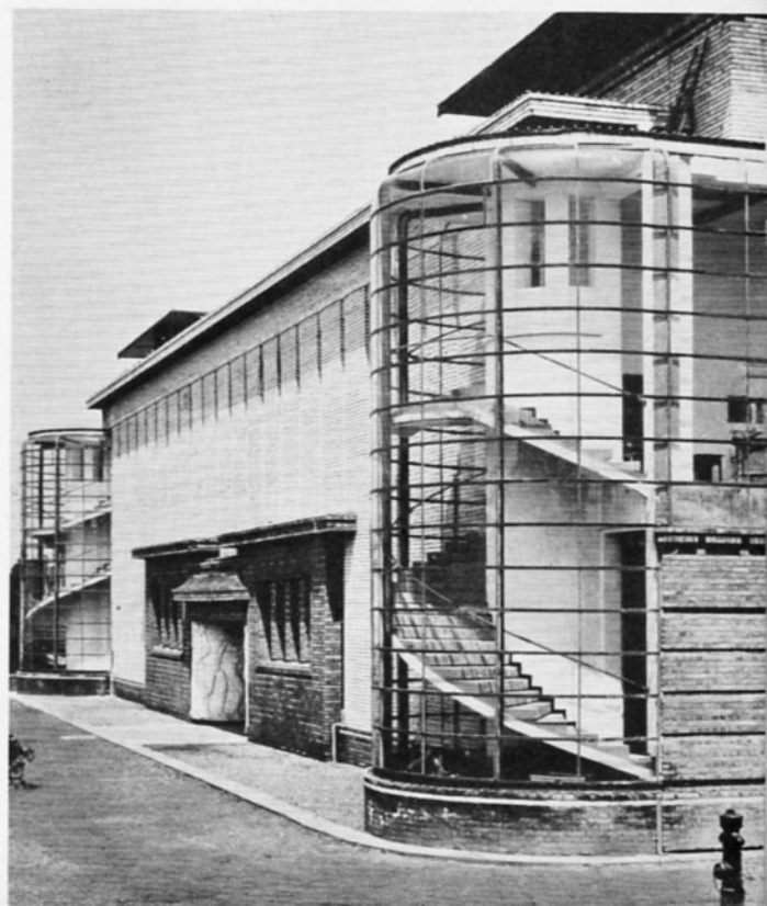
Walter Gropius and Adolf Meyer: Cologne Exposition of the German Werkbund. Administration Building. Front view. 1914
