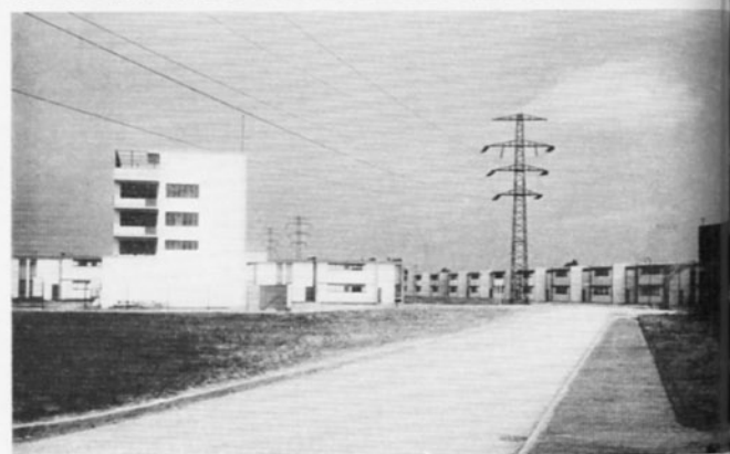
Walter Gropius: Dessau-Törten, a community of workers' houses. General view. 1926
