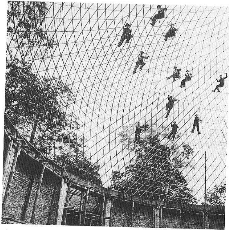
Planetarium under construction in Jena in the 1920s
