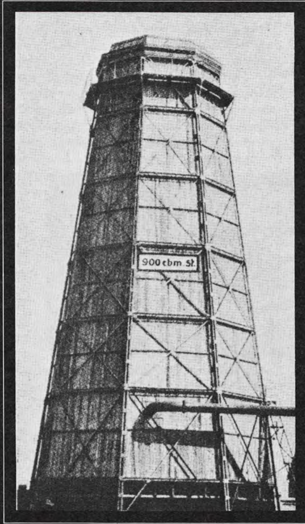
Steam cooler for the Tissen machine factory
