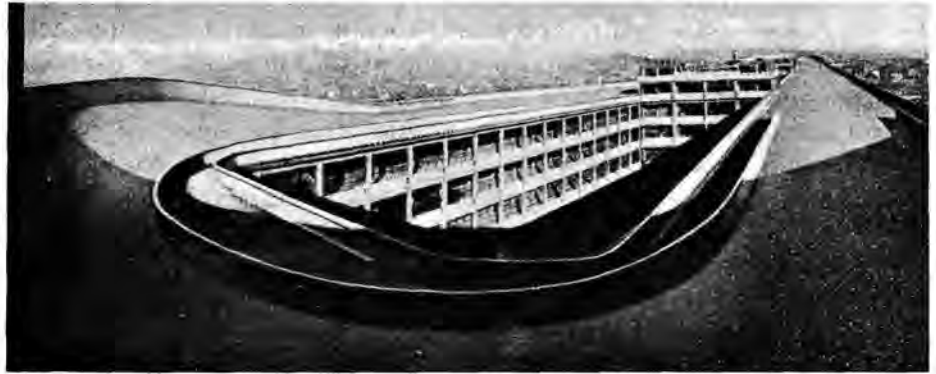
Testing track on the roof of the Fiat automobile factory in Turin
