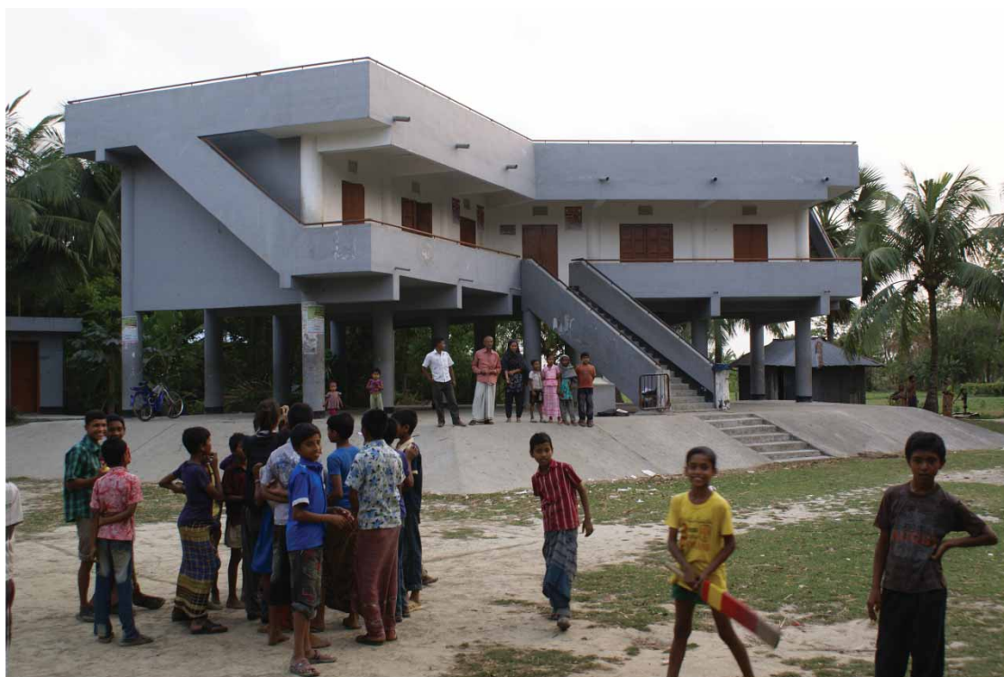
Existing cyclone shelter, Rangabali, photo: Lindsay Bremner
