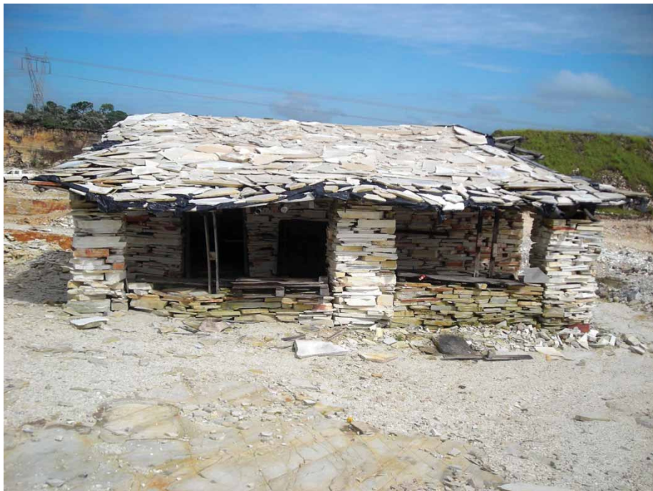
Images from inspection reports compiled by the Brazilian Ministry of Work and Employment: workers' transport and accommodation, Minas Gerais, Brazil
