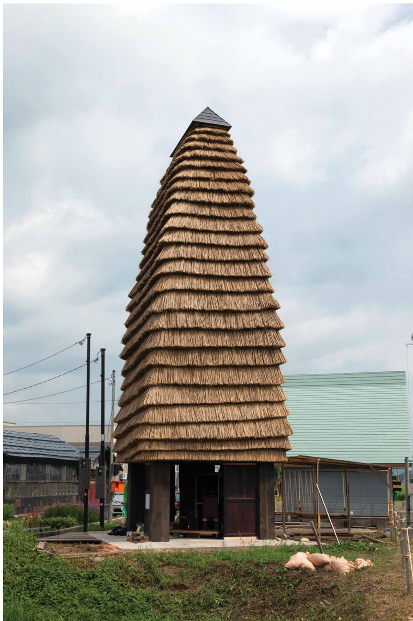
MIKAN + Sogabe Lab, Kanagawa University, Gejo Thatch Tower , Echigo-Tsumari Art Triennale 2012, wood, thatch, old tools and furnitures etc, approx 12m tall, floor space 8 square meter, photo courtesy Osamu Nakamura
