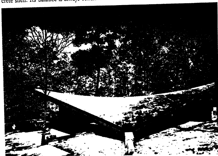
64. Eduardo F. Catalano: House at Raleigh, N.C., 1955. The hyperbolic paraboloid has the same significance whether constructed of wood or as a concrete shell. Its balance is always contained within itself.
