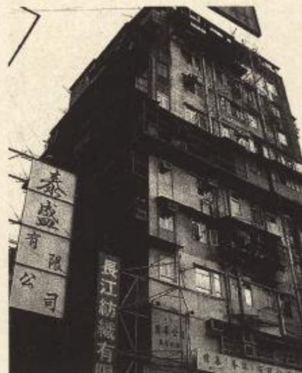
Illegal facades, Hong Kong
